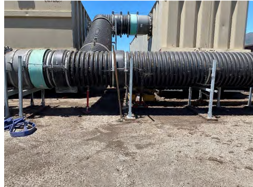
Photograph 29B. July 14, 2023. There is no longer wastewater below the conveyance system.
