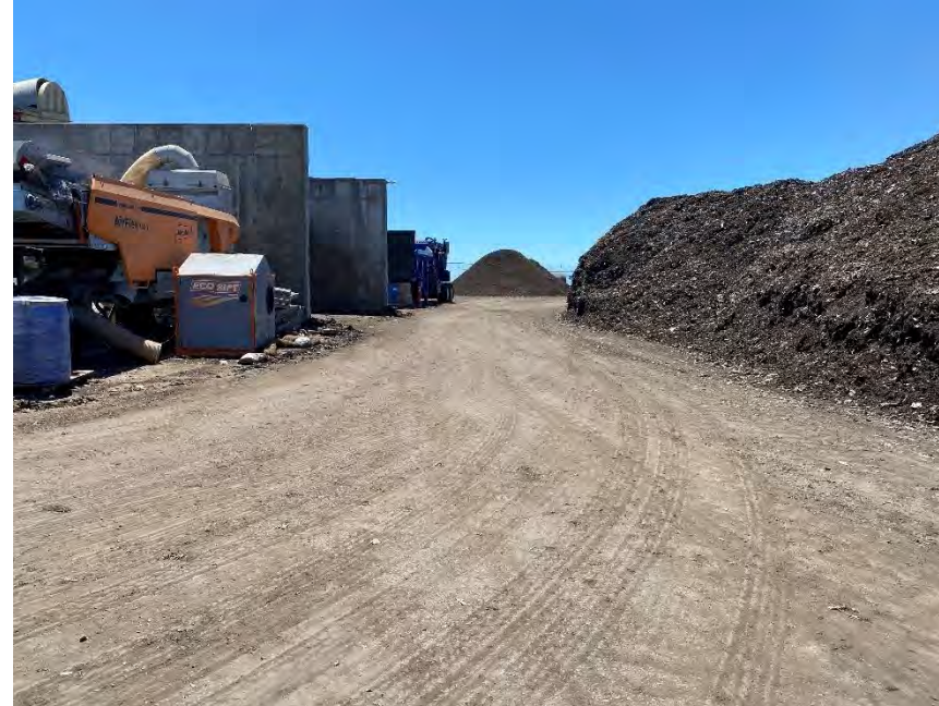
Photograph 22B. July 14, 2023. The working surface where feedstock/ digestate enters the facility from ADF has been repaired with asphalt.
