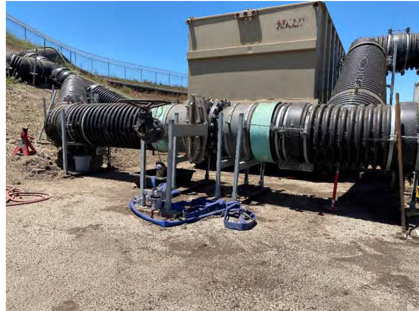
Photograph 30B. July 14, 2023. There is no longer wastewater below the conveyance system.
