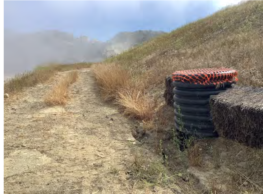
Photograph 34B. July 11, 2023. Stained soil has been removed and stored in a roll off bin.
