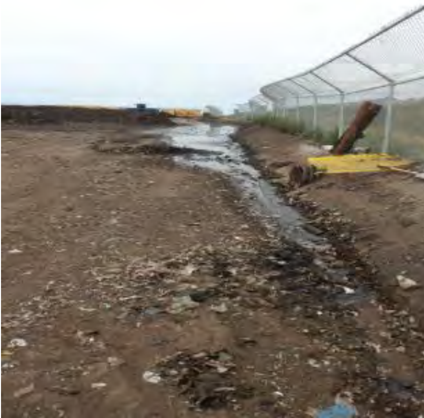
Photograph 6A. June 13, 2023. Pondered wastewater at the northern portion of the working surface.
