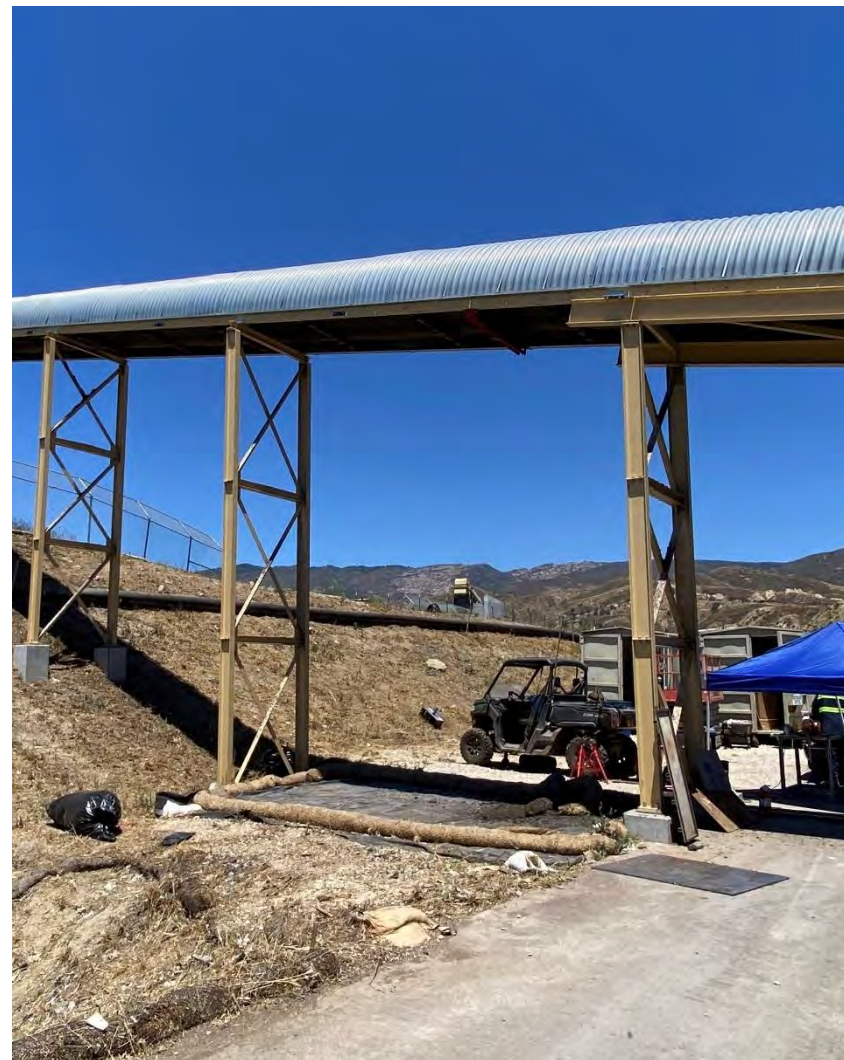
Photograph 1B. July 14, 2023. Scraper pending installation on conveyor belt.
