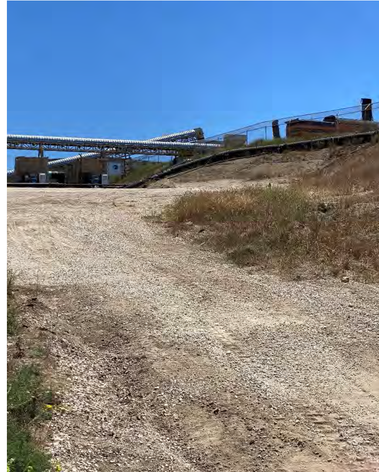
Photograph 33B. July 14, 2023. Stained soil has been removed and stored in a roll off bin.
