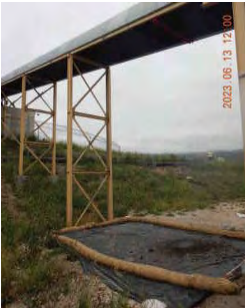
Photograph 1A. June 13, 2023. Conveyor system that moves compost feedstock (digestate) from the ADF to the CMU continues to have feedstock material beneath the conveyor from fallen material.
