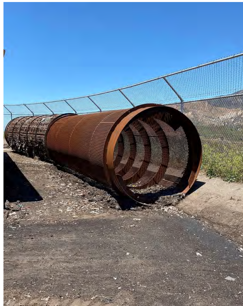
Photograph 13B. July 14, 2023. No water observed.
