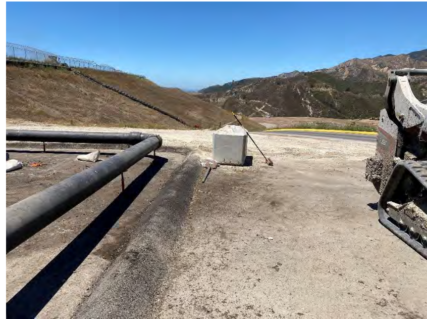
Photograph 23B. July 14, 2023. An asphalt berm has been installed to prevent discharge.
