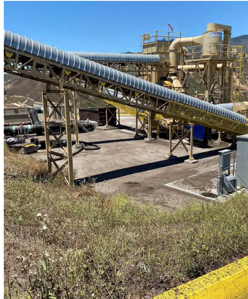
Photograph 2B. July 14, 2023. Asphalt berm has been installed to the west side of the baker tanks.
