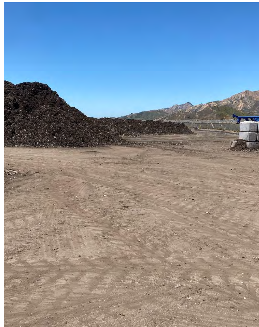
Photograph 11B. July 14, 2023. Damaged areas of the working surface have been repaired with asphalt.
