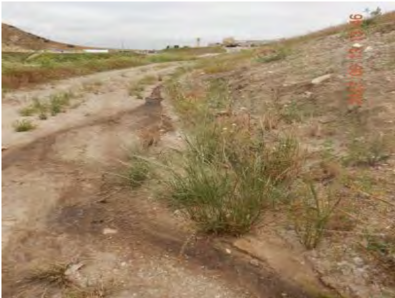
Photograph 35A. June 13, 2023. Wastewater flowing along landfill bench over an unlined area of the landfill.
