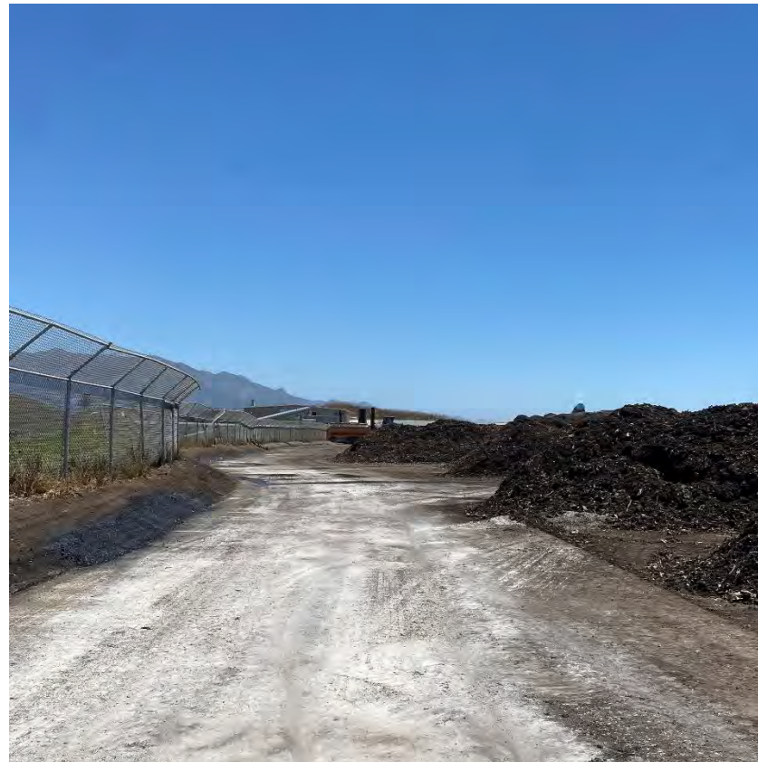
Photograph 12B. July 14, 2023. Pondered water was not observed at the northern portion of the facility. Storm drain inlets have been blocked to prevent discharge to the conveyance system.
