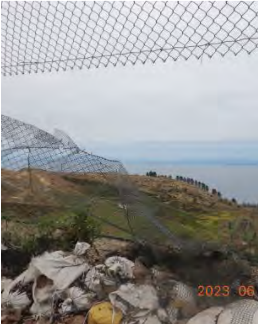
Photograph 18A. June 13, 2023. Damaged litter fence.
