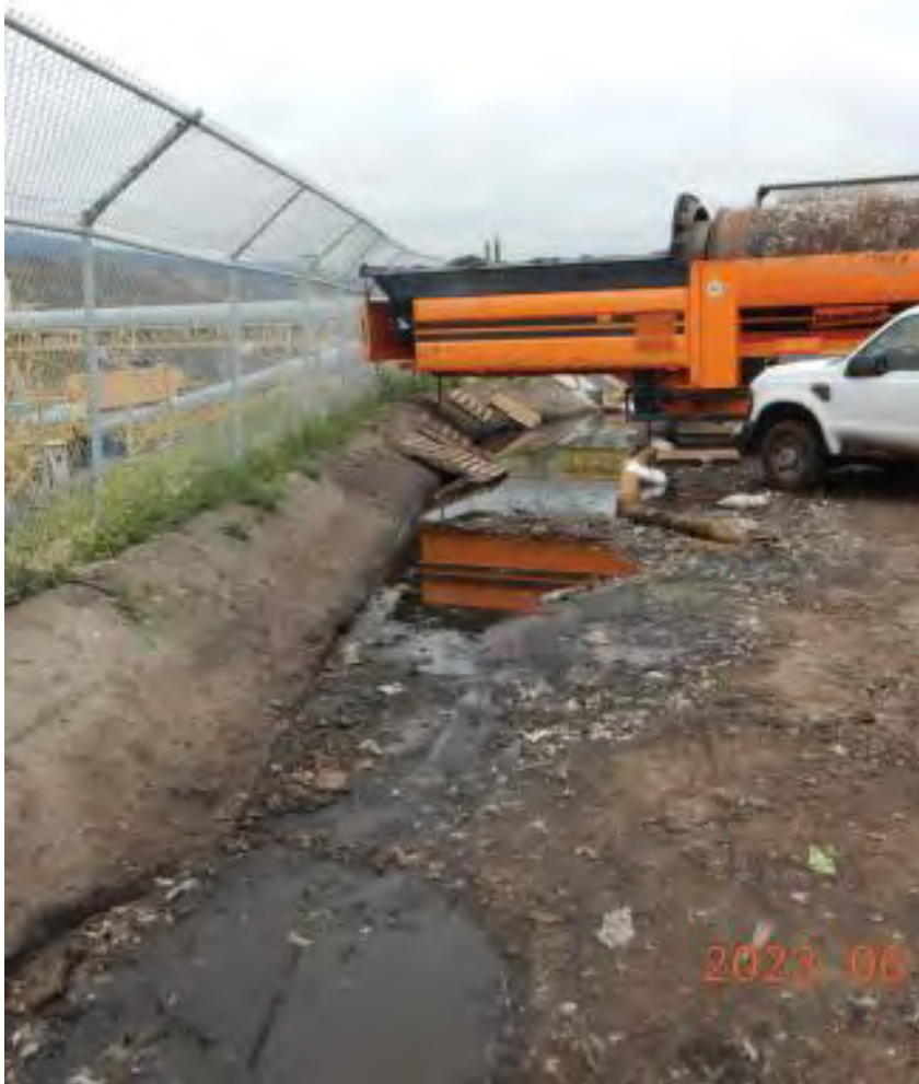
Photograph 4A. June 13, 2023. Pondered wastewater near the north area of the working surface and at the stormwater/wastewater outlet to the stormwater/ wastewater conveyance pipes.
