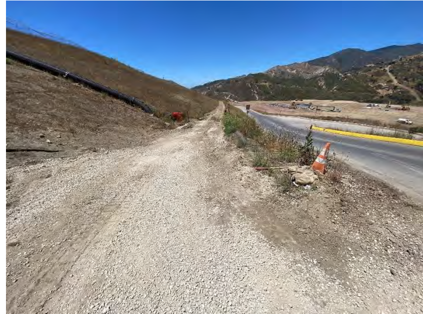
Photograph 31B. July 14, 2023. Stained soil has been removed and stored in a roll off bin.
