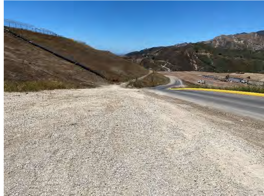
Photograph 26B. July 14, 2023. Stained soil has been removed and stored in a roll off bin.
