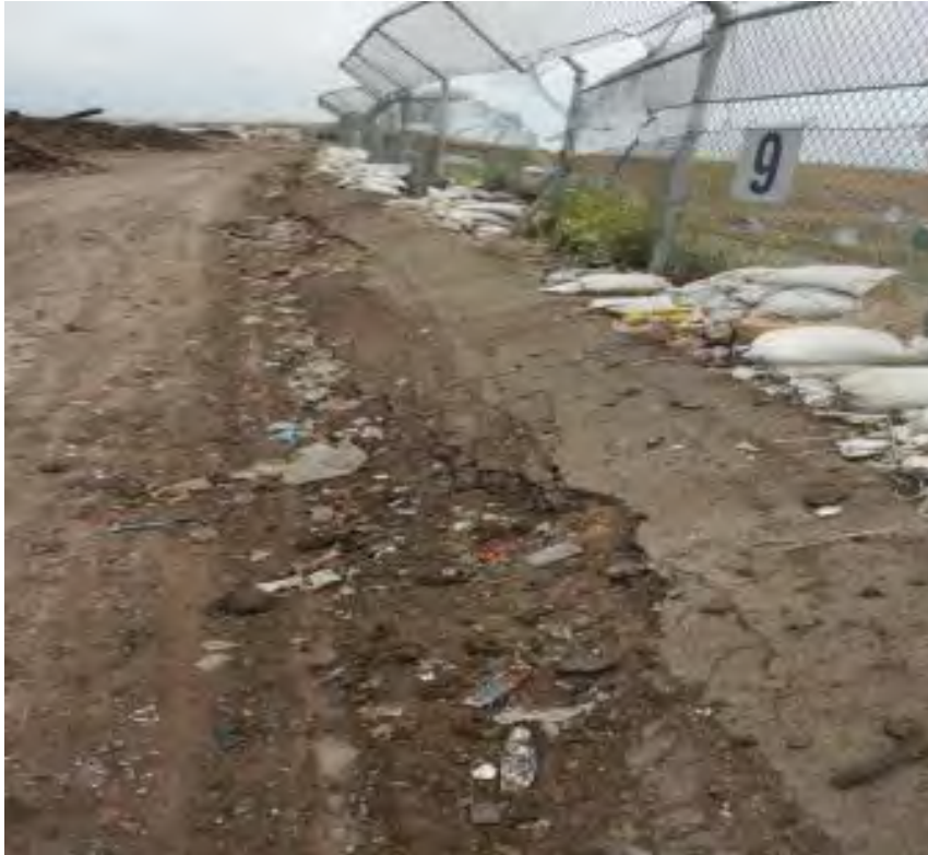
Photograph 17A. June 13, 2023. Damaged working surface, berms, and litter fence.
