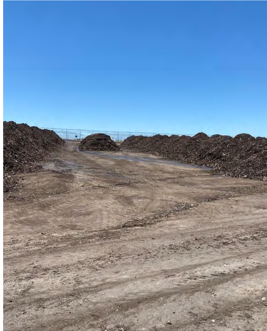
Photograph 7B. July 14, 2023. Compost windrows. Minimal leachate observed.
