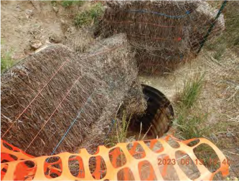
Photograph 32A. June 13, 2023. Pipe on bench where wastewater flows to the landfill north sediment basin.
