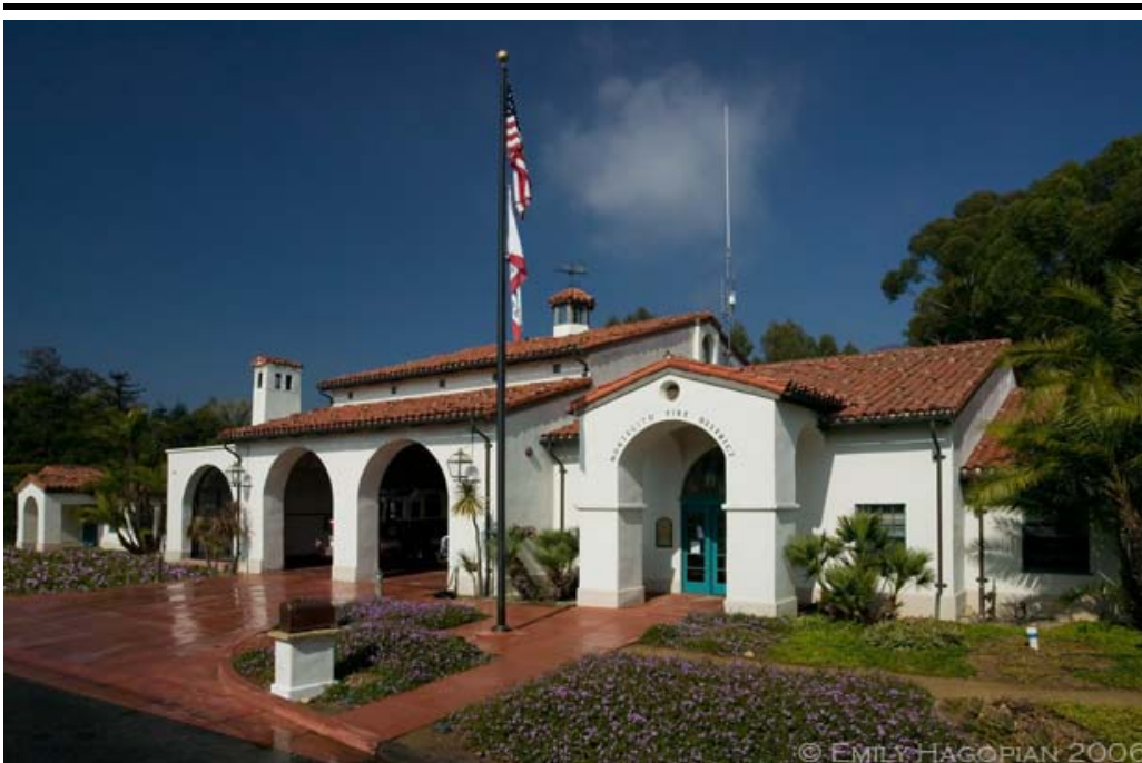
Montecito Fire Station #1. Source: MFPD
