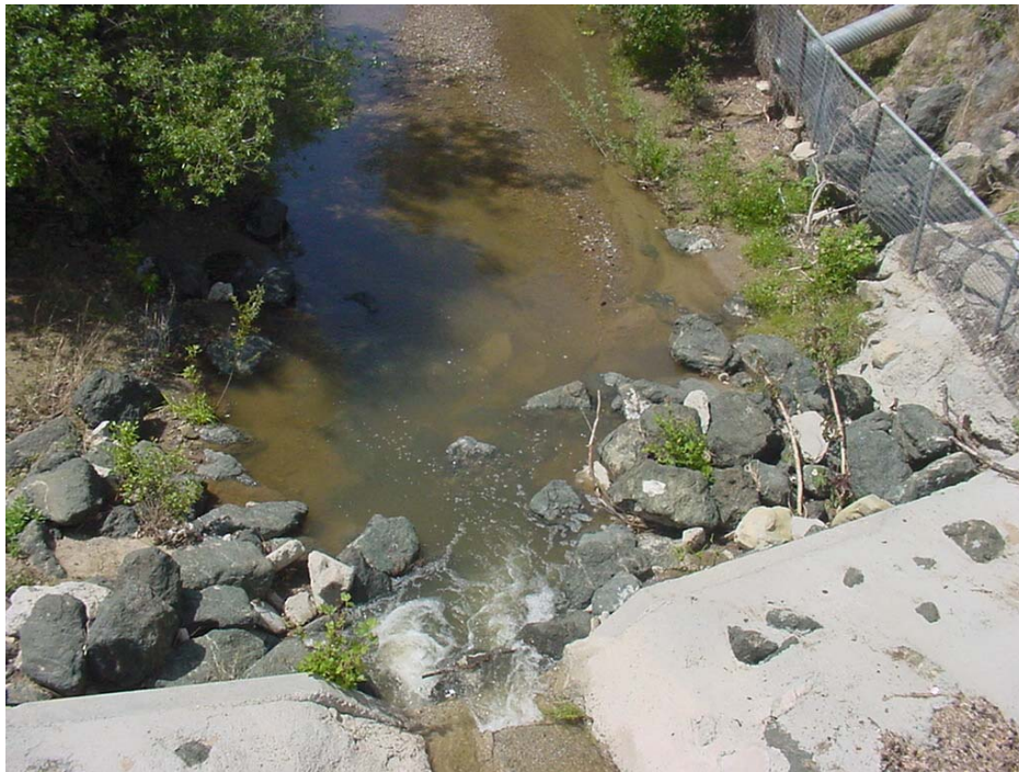
Existing Conditions: Maria Ygnacio Creek at Hollister Bridge 51C-026
