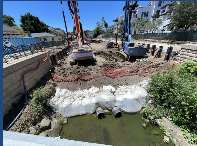
Lower Mission Creek Reach 4 Construction
