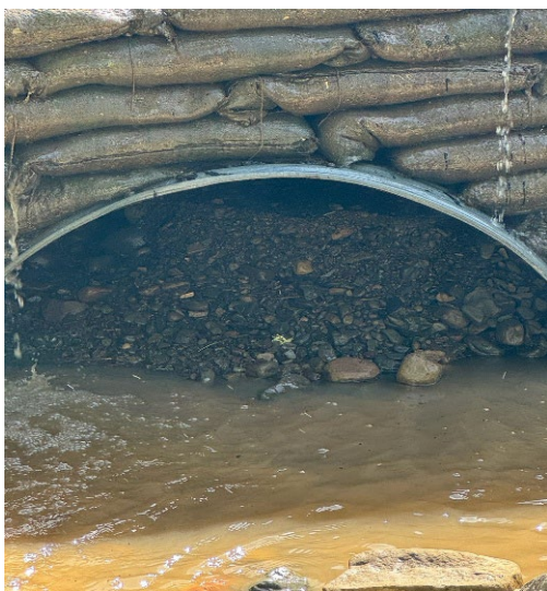
Figure 1: Debris blocking existing culvert
