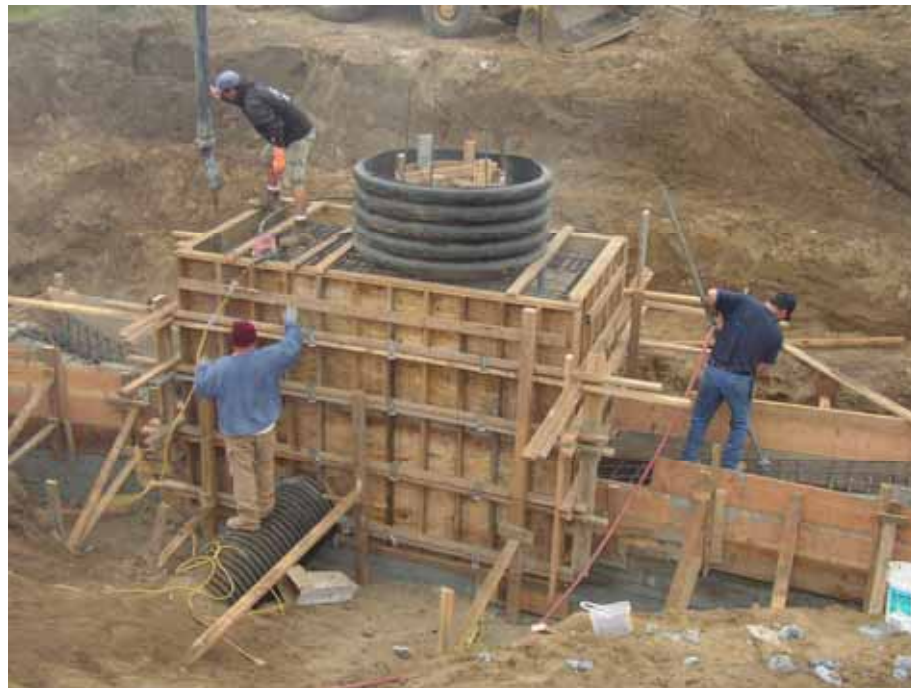
Getty/Kovar/Hobbs Interconnect Project Construction
