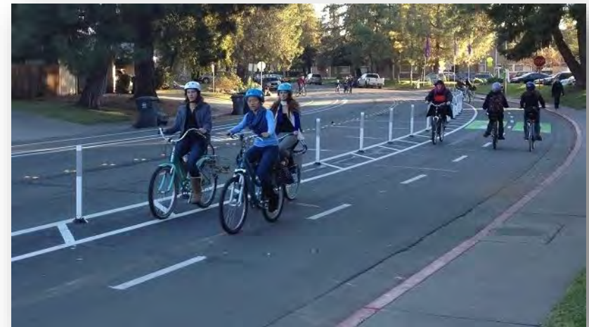
Class IV Bikeways offer a protected right-of-way, separate from street traffic. Image Source: Sacramento Area Council of Governments. ( https://www.sacog.org/post/class-iv-bikeways )
