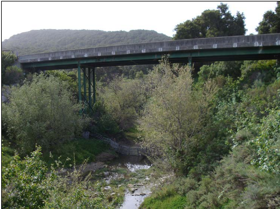
Jalama Road Bridge, view to the southeast
