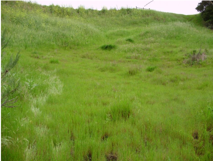
Photo 3. Seep area on eastern bank of Jalama Creek, in a rotational landslide.
