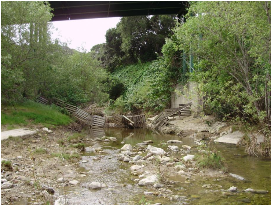
Photo 2. View of Jalama Creek from north of Bridge 17. Note the cattle exclusion draped across the creek at the bridge.
