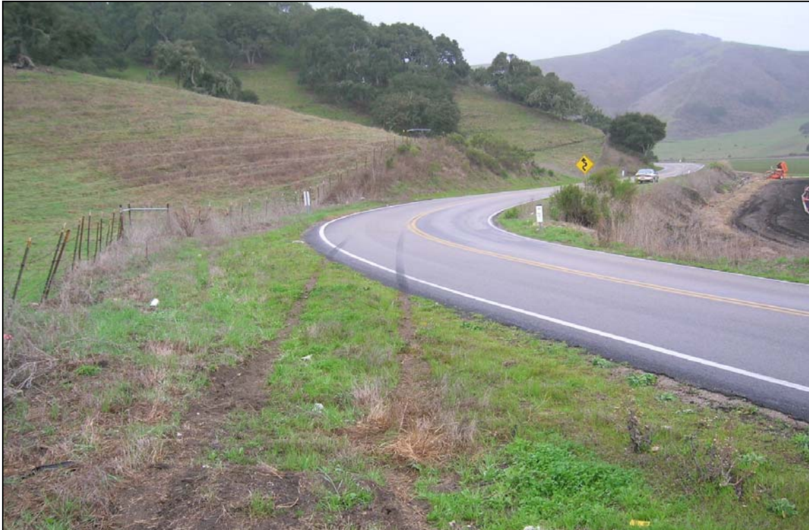
Harris Grade HR3 Improvement Project Site
