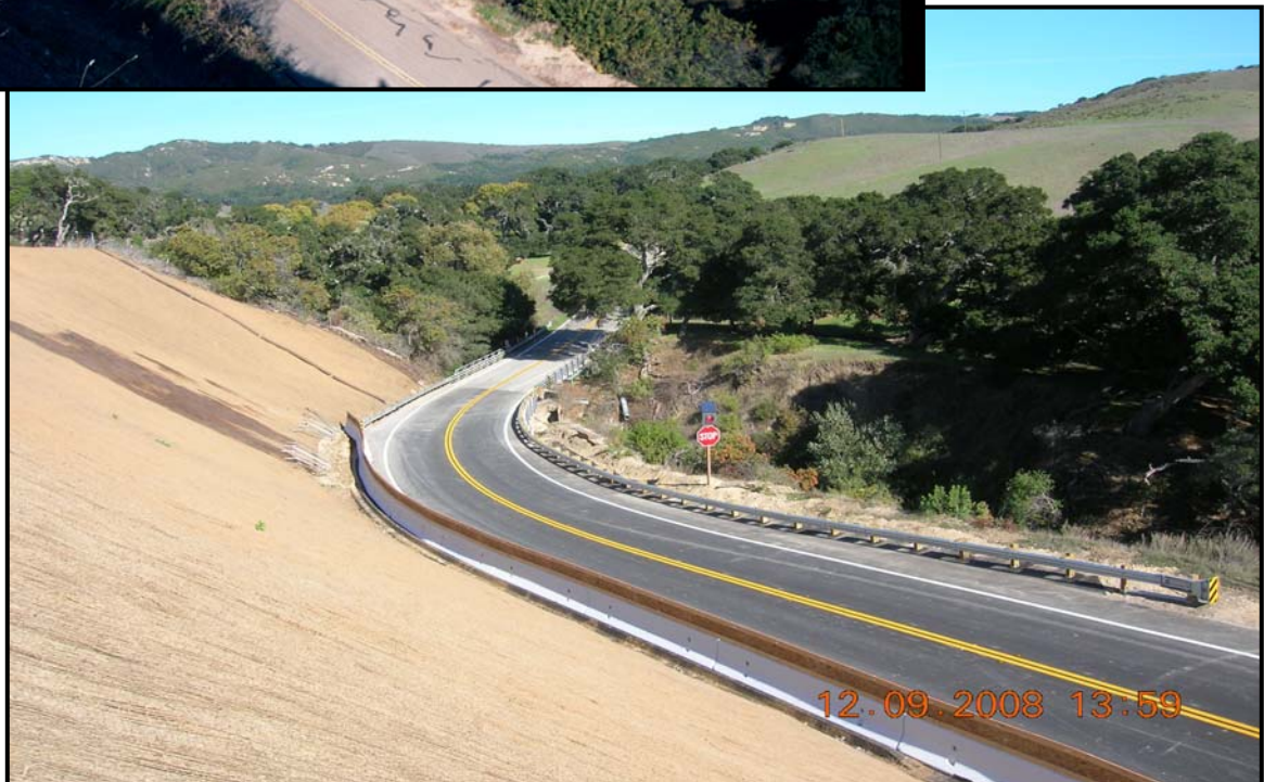
Jalama Road Three Days Prior to Project Completion
