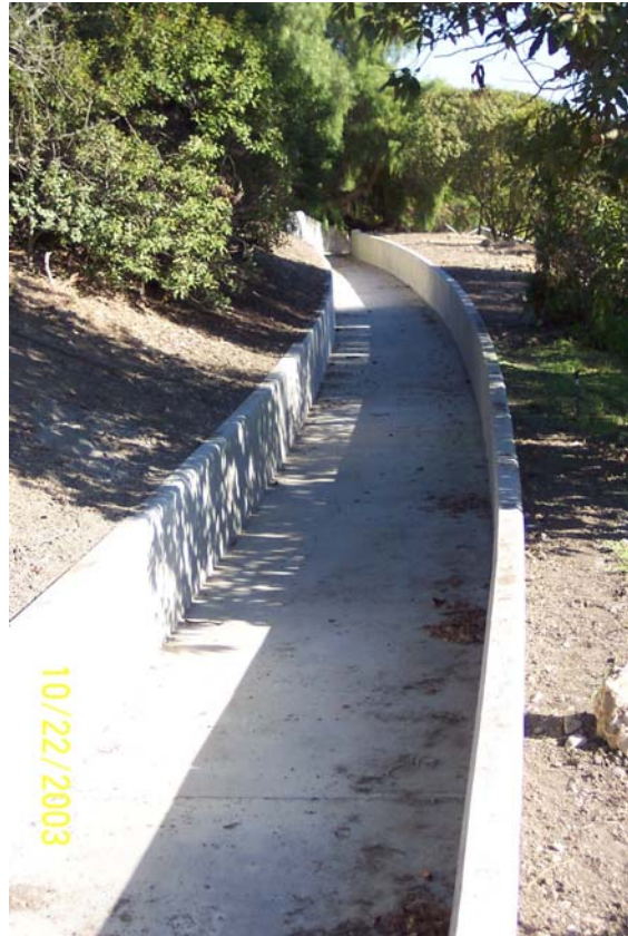
Serenidad Interceptor Channel Project Completion
