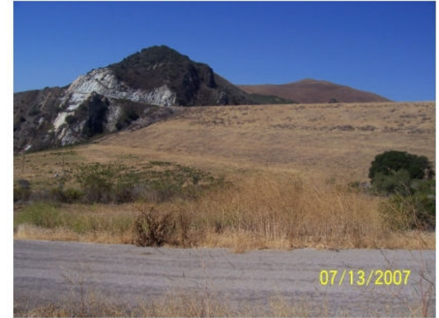
Twitchell Earth-Filled Dam
