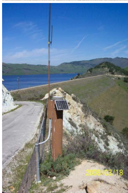
Figures 75 & 76 – Twitchell Reservoir & Dam
