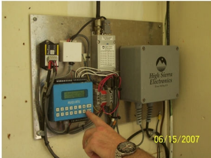
Water Level & Gate Opening ALERT Instrumentation (RUG3)
