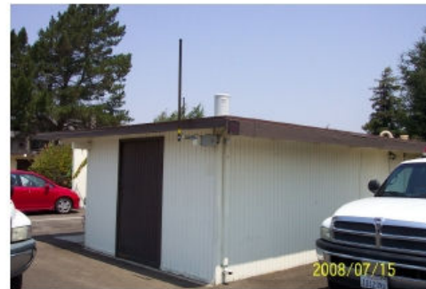
ALERT 0.01" Rooftop Install (Buellton Fire)
