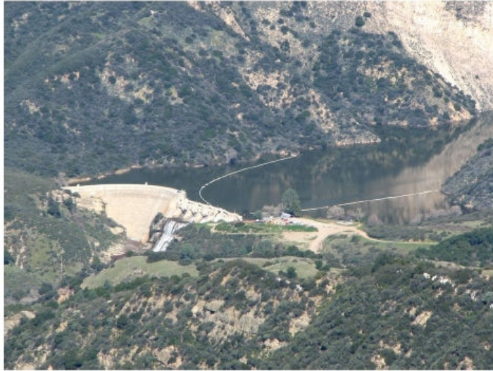
Gibraltar Reservoir & Dam
