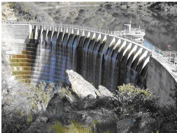
Figure 72 – Juncal Dam & Spillway
