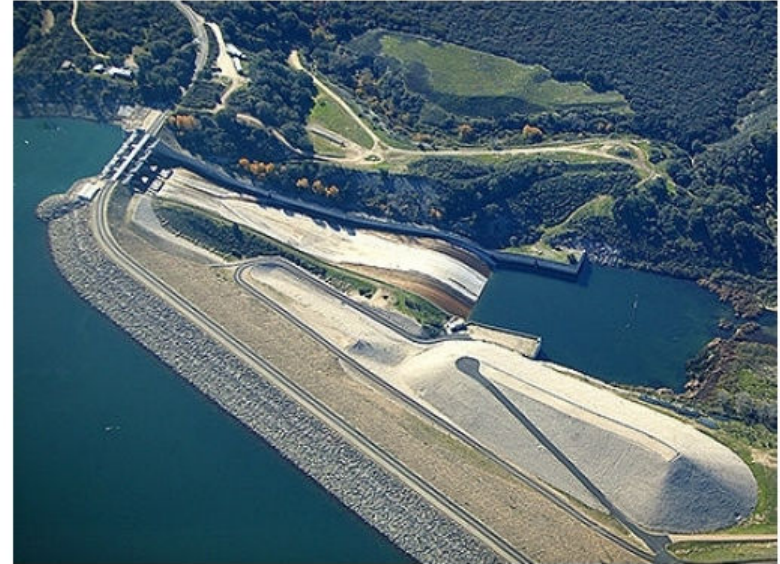
Bradbury Dam & Spillway
