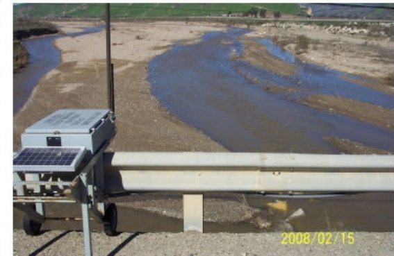
ALERT Radar (Sisquoc River @ Garey)
