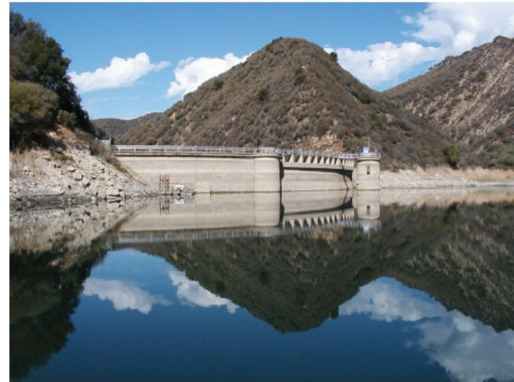
Jameson Reservoir & Dam
