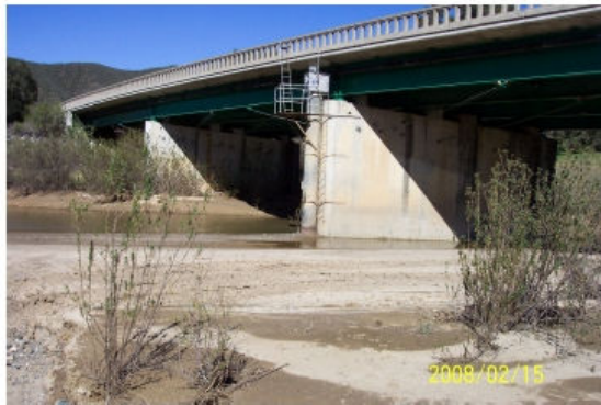
ALERT Bubbler (Cuyama River @ Buckhorn)
