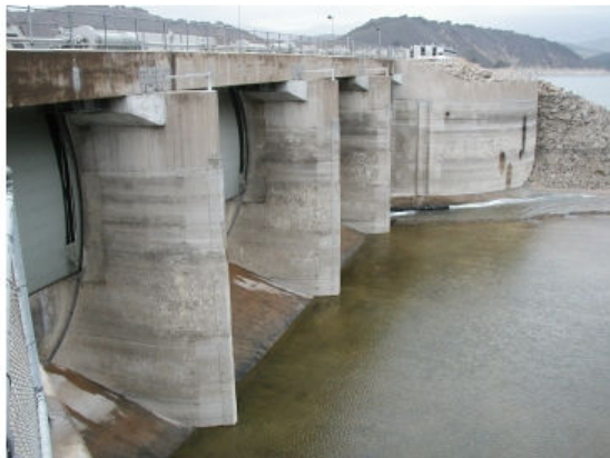
Bradbury Dam Gates
