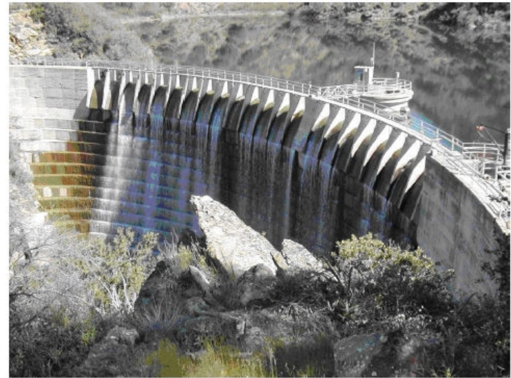
Jameson Dam & Spillway
