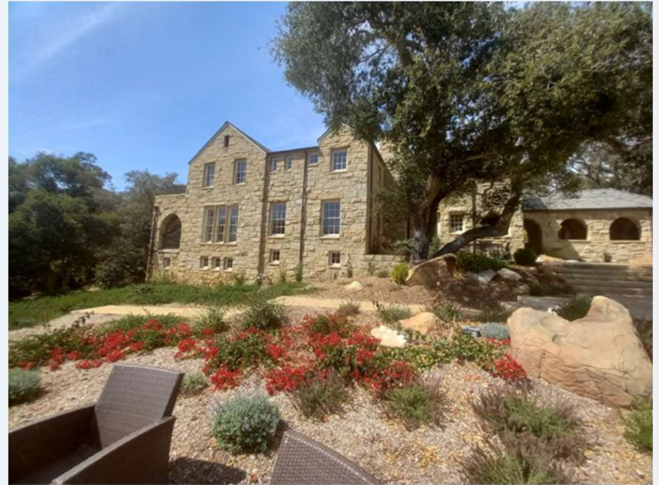
Residence, south elevation, looking north
