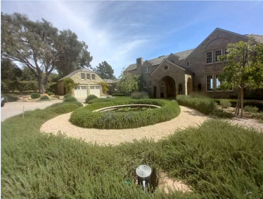
Residence, garage, and motor court, looking southeast
