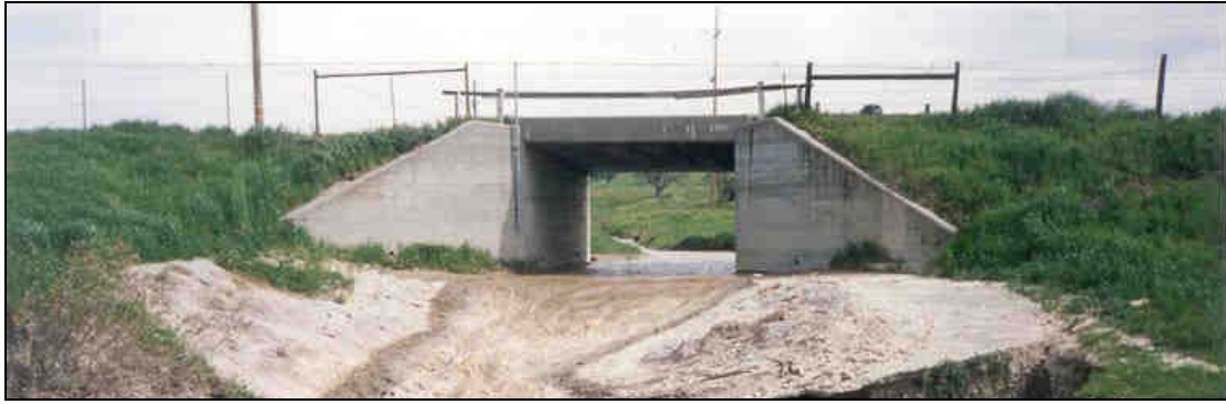
Zaca Station Road Bridge No. 51C-087, looking north
