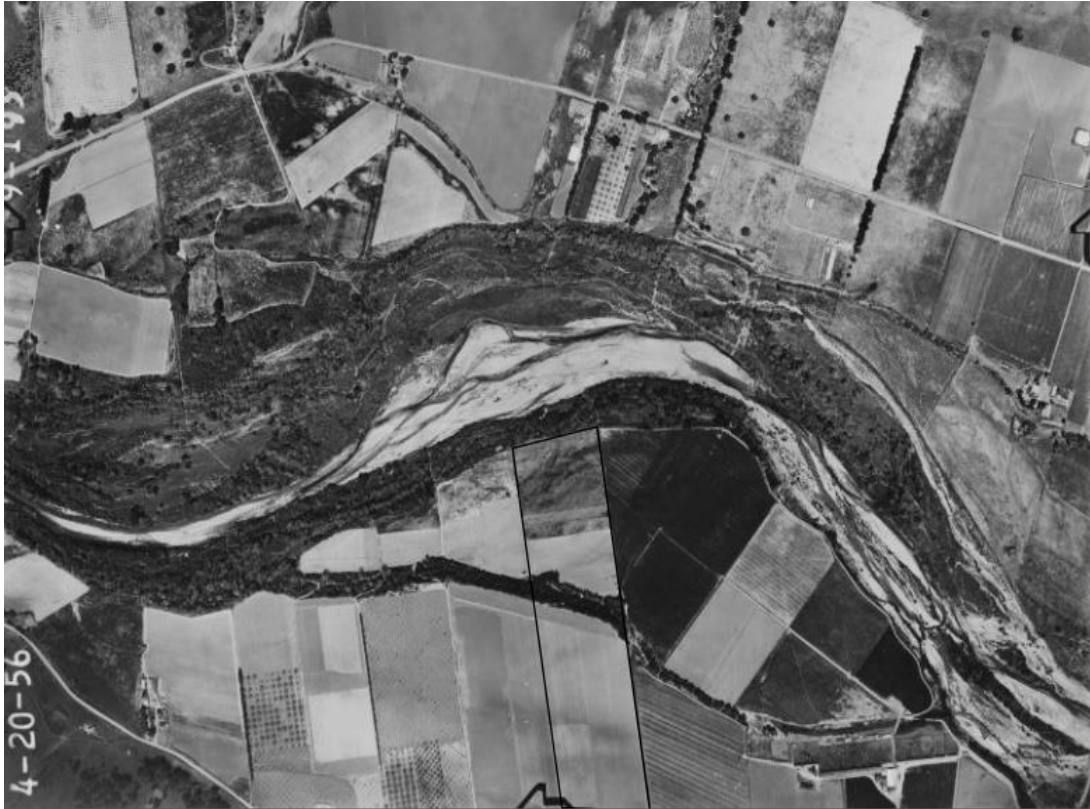
Photograph 3. Historic imagery of project site; April 20, 1956 (UCSB 2020)
