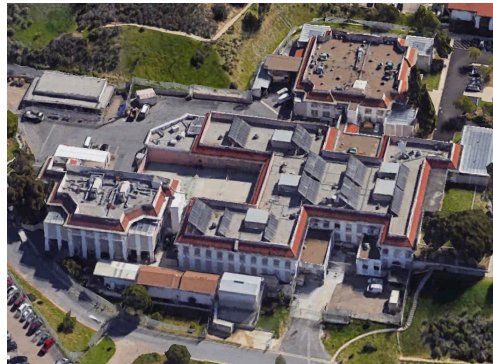
SB Main Jail Renovation
