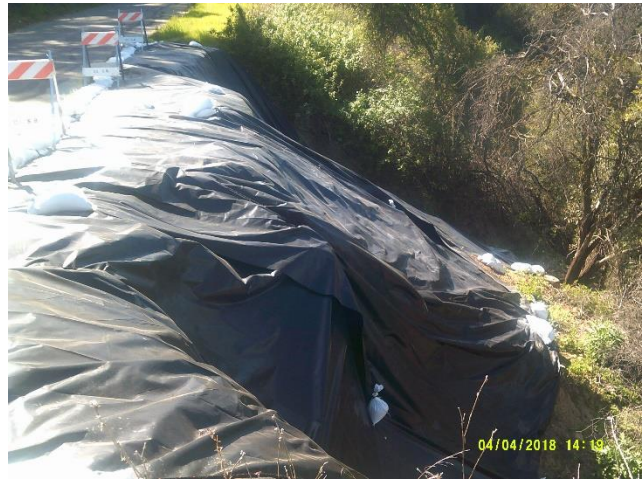
862414 Tepusquet Road MP 11. Looking North. Failed roadway support embankment and landslide scarp shown in left photo. Temporary Erosion Control Measures shown in right photo.
