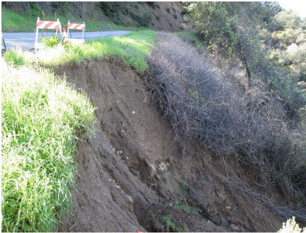
862414 Tepusquet Road MP 11. Looking North. Failed roadway support embankment and landslide scarp shown in left photo. Temporary Erosion Control Measures shown in right photo.
