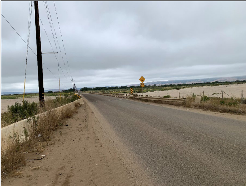
c. Bridge approach roadway from the north, facing south
