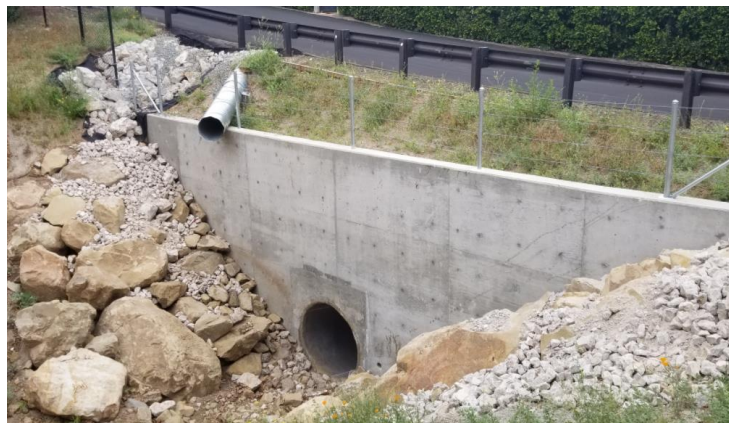
Figure 2: 2018 Storm Damage Repair on Brooktree Road and Culvert Replacement
