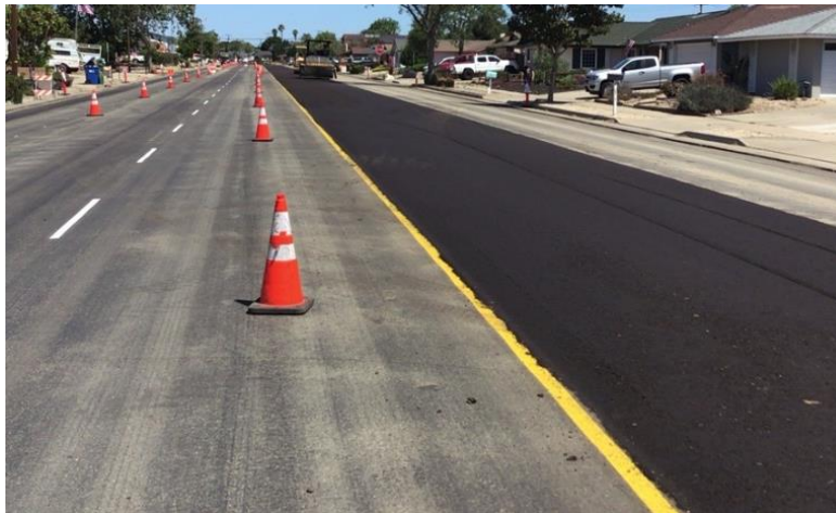
Figure 3: Constellation Road Pavement Rehabilitation
