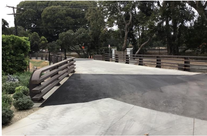
Figure 1: Fernald Point Lane Bridge Replacement, New Bridge No. 51C-0362
