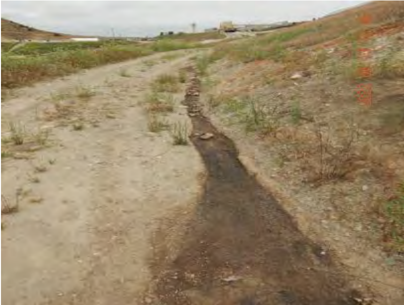
Photograph 36A. June 13, 2023. Wastewater flowing along landfill bench over an unlined area of the landfill.
