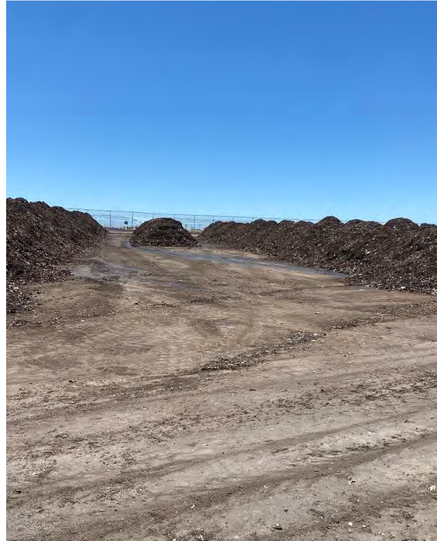
Photograph 10B. July 14, 2023. CMU deck has been allowed to dry.
