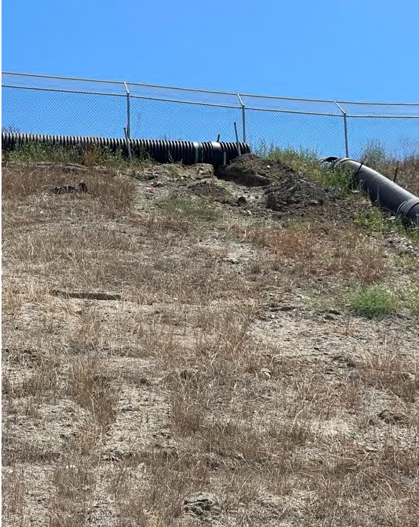
Photograph 3. View facing southwest.
