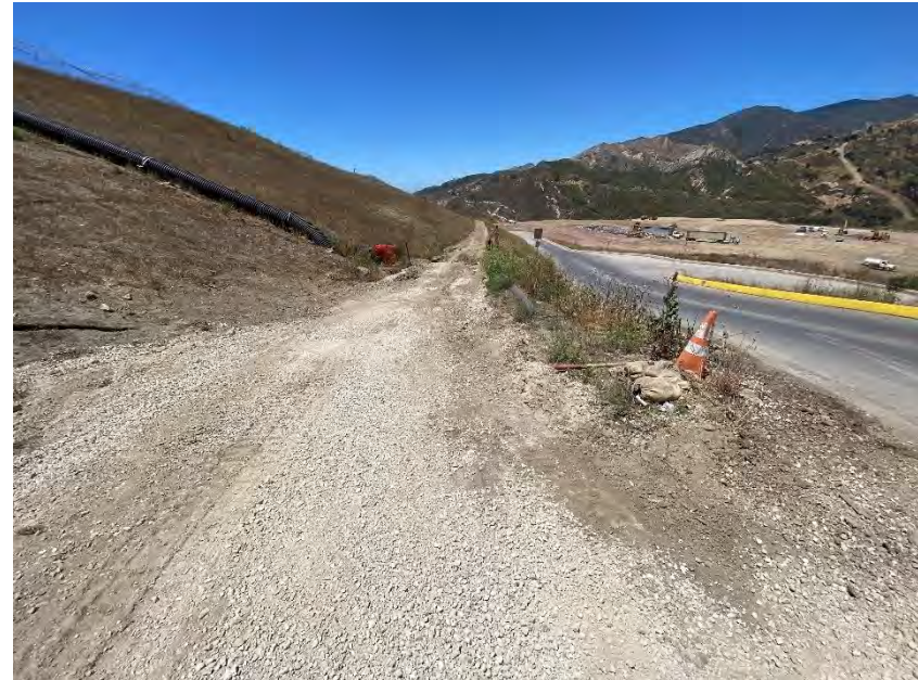
Photograph 31B. July 14, 2023. Stained soil has been removed and stored in a roll off bin.
