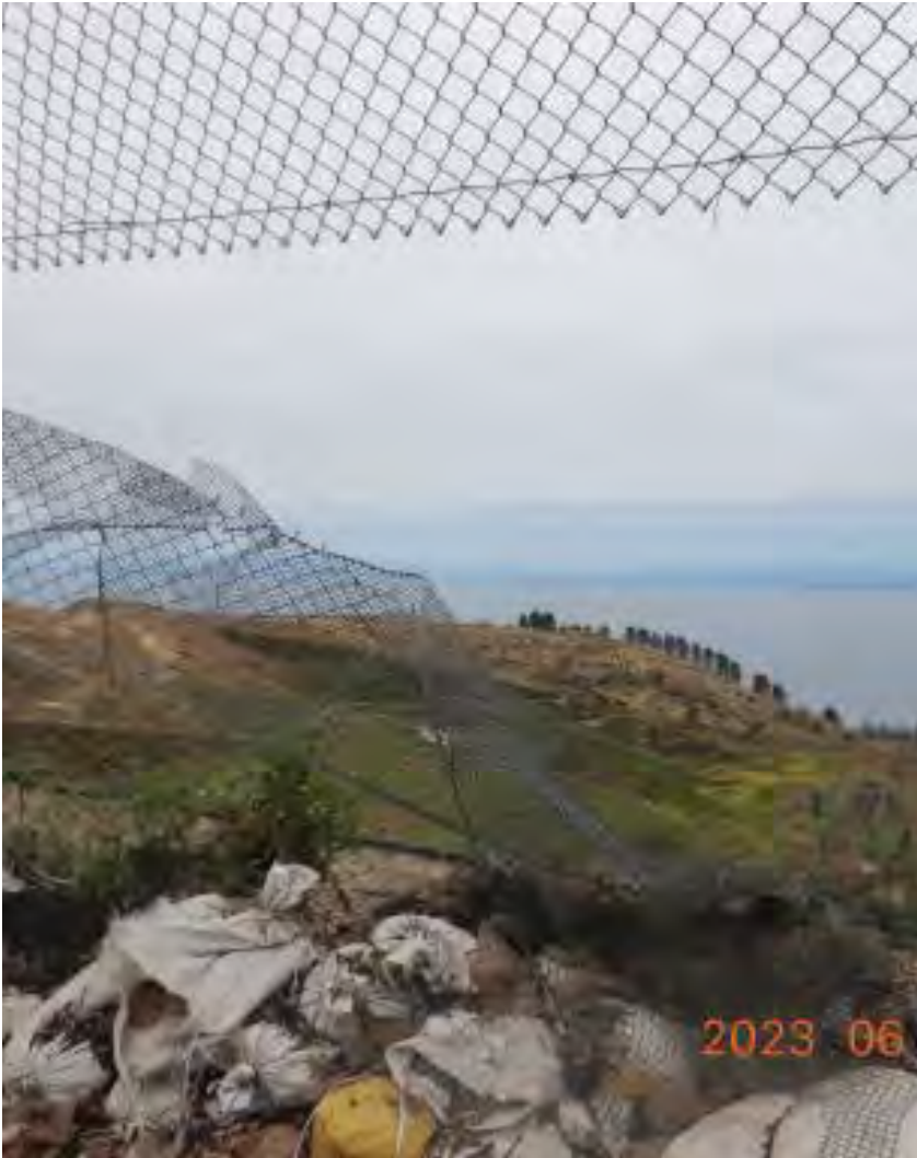
Photograph 18A. June 13, 2023. Damaged litter fence.
