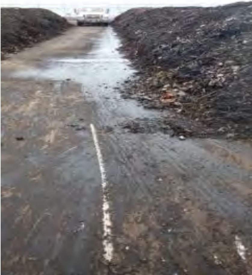
Photograph 11A. June 13, 2023. Damaged area of the working surface with ponded water and scraped asphalt surface.
