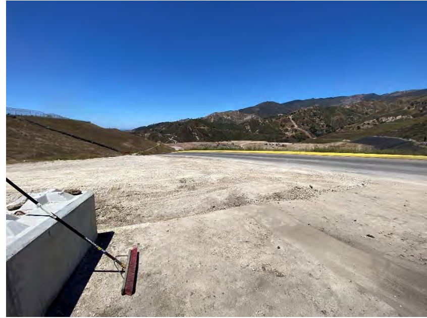
Photograph 24B. July 14, 2023. An asphalt berm has been installed to prevent discharge.
