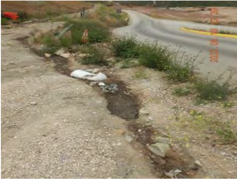
Photograph 31A. June 13, 2023. Wastewater flowing from the D-table area towards a lower landfill bench.
