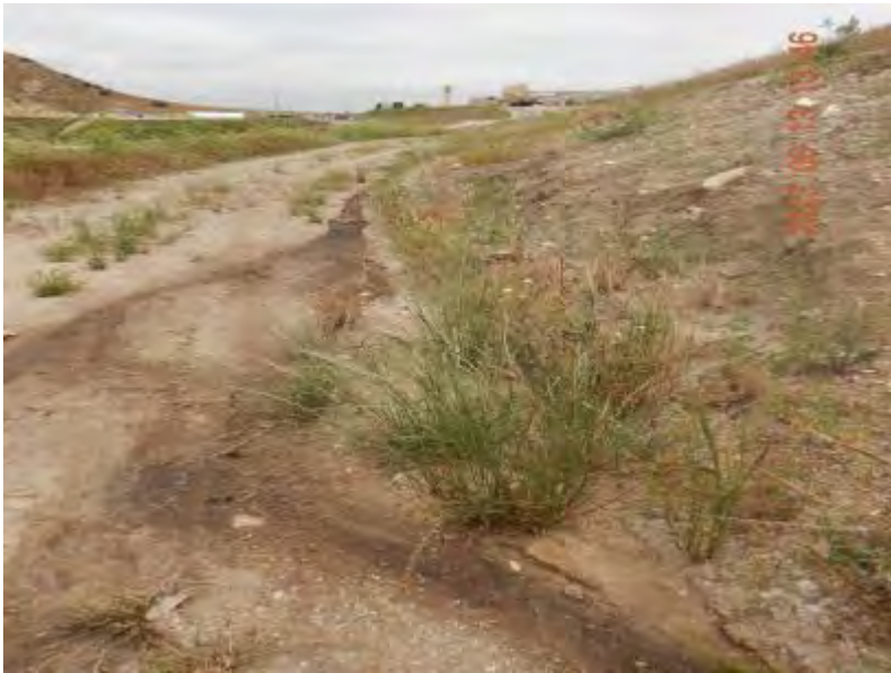
Photograph 35A. June 13, 2023. Wastewater flowing along landfill bench over an unlined area of the landfill.
