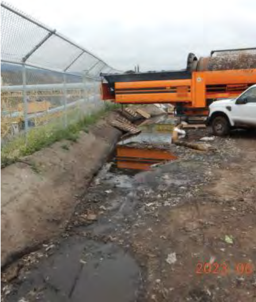
Photograph 4A. June 13, 2023. Pondered wastewater near the north area of the working surface and at the stormwater/wastewater outlet to the stormwater/ wastewater conveyance pipes.
