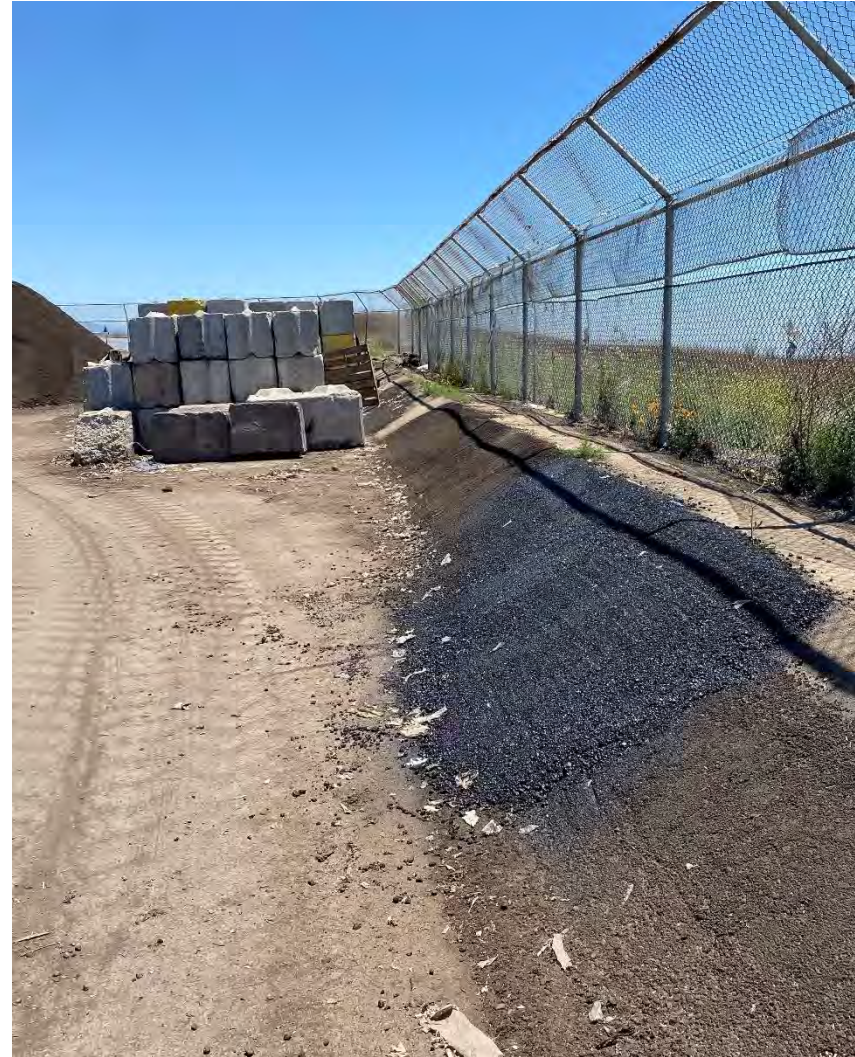
Photograph 20B. July 14, 2023. The facility berm has been repaired with asphalt.
