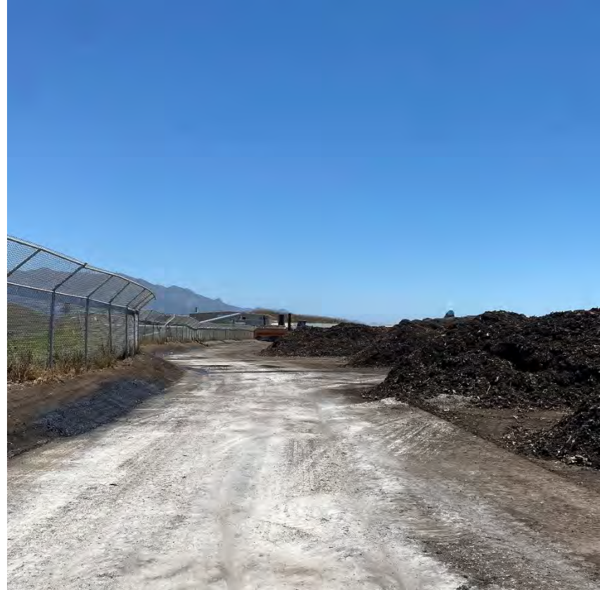
Photograph 12B. July 14, 2023. Pondered water was not observed at the northern portion of the facility. Storm drain inlets have been blocked to prevent discharge to the conveyance system.
