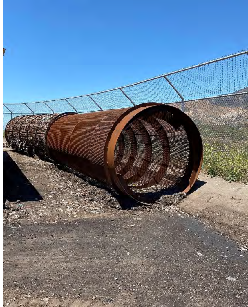
Photograph 13B. July 14, 2023. No water observed.
