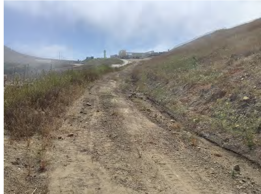
Photograph 35B. July 11, 2023. Stained soil has been removed and stored in a roll off bin.
