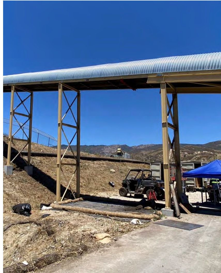
Photograph 1B. July 14, 2023. Scraper pending installation on conveyor belt.
