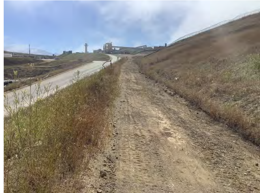
Photograph 36B. July 11, 2023. Stained soil has been removed and stored in a roll off bin.
