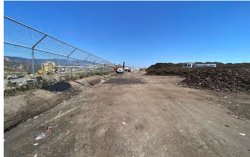
Photograph 8. View facing northeast.
