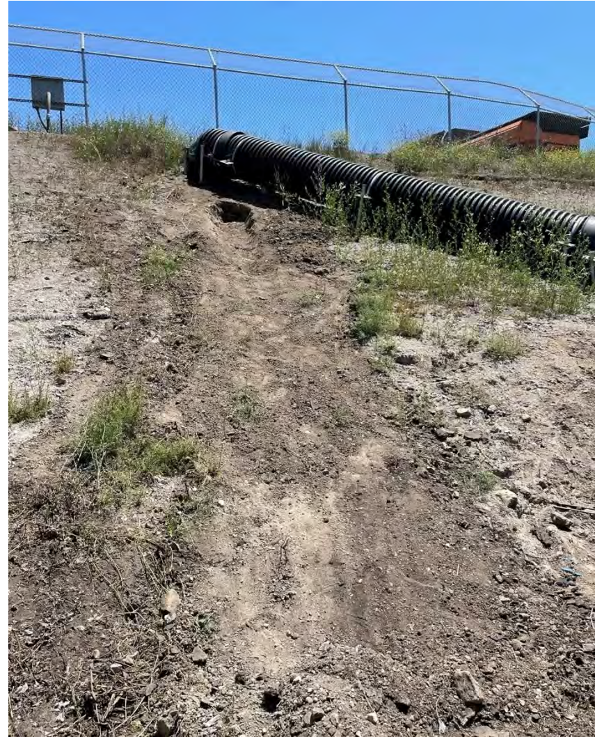
Photograph 8. View facing southwest.
