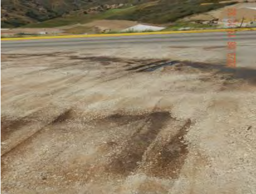
Photograph 25A. June 13, 2023. Wastewater outside of the working surface within recently placed gravel.
