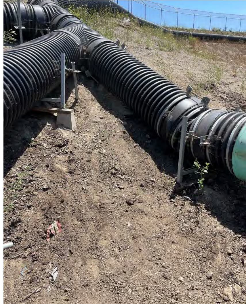
Photograph 6. View facing southwest.
