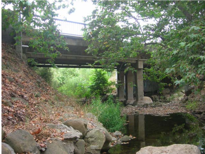
Cathedral Oaks Road Bridge (No. 51C-001) at San Antonio Creek
