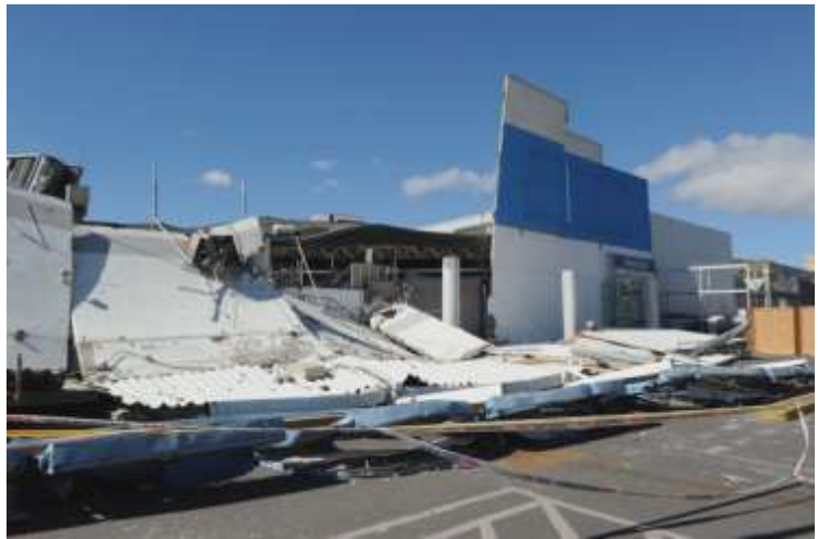
Tilt-up Building Collapse
