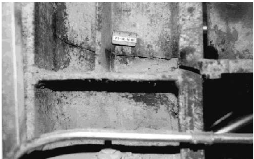
Steel Moment Fracture Due to Earthquake
