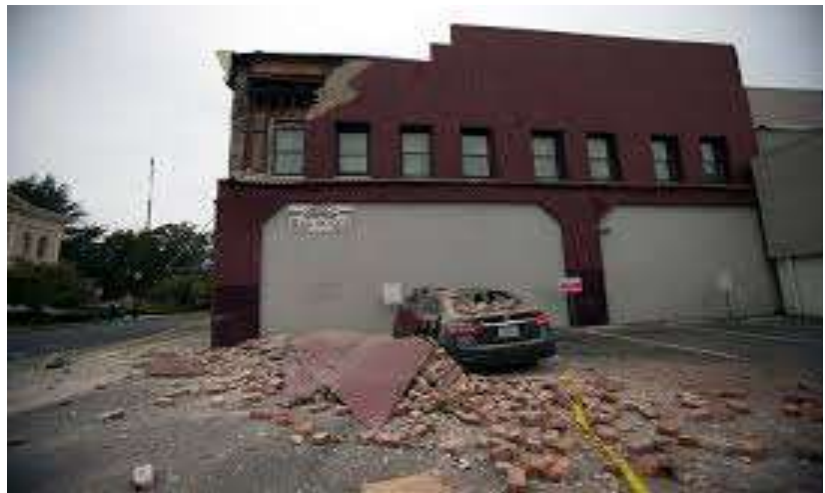
Failure of URM Building
