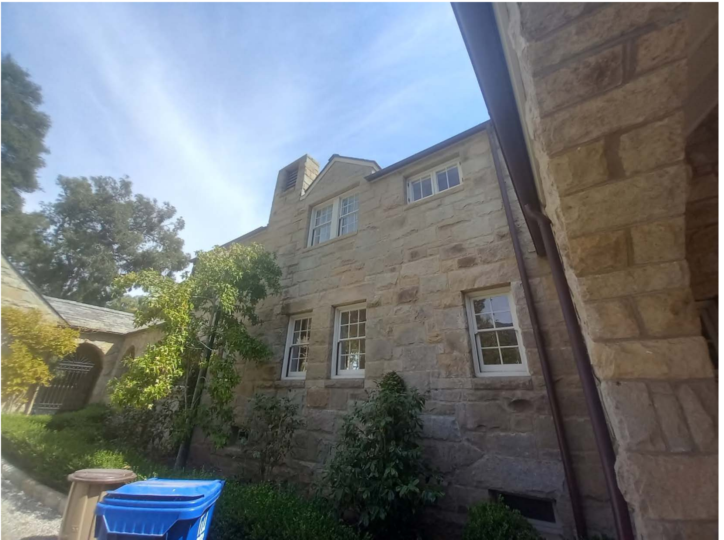
Photograph 5, Residence, east end of the north elevation, looking southeast
