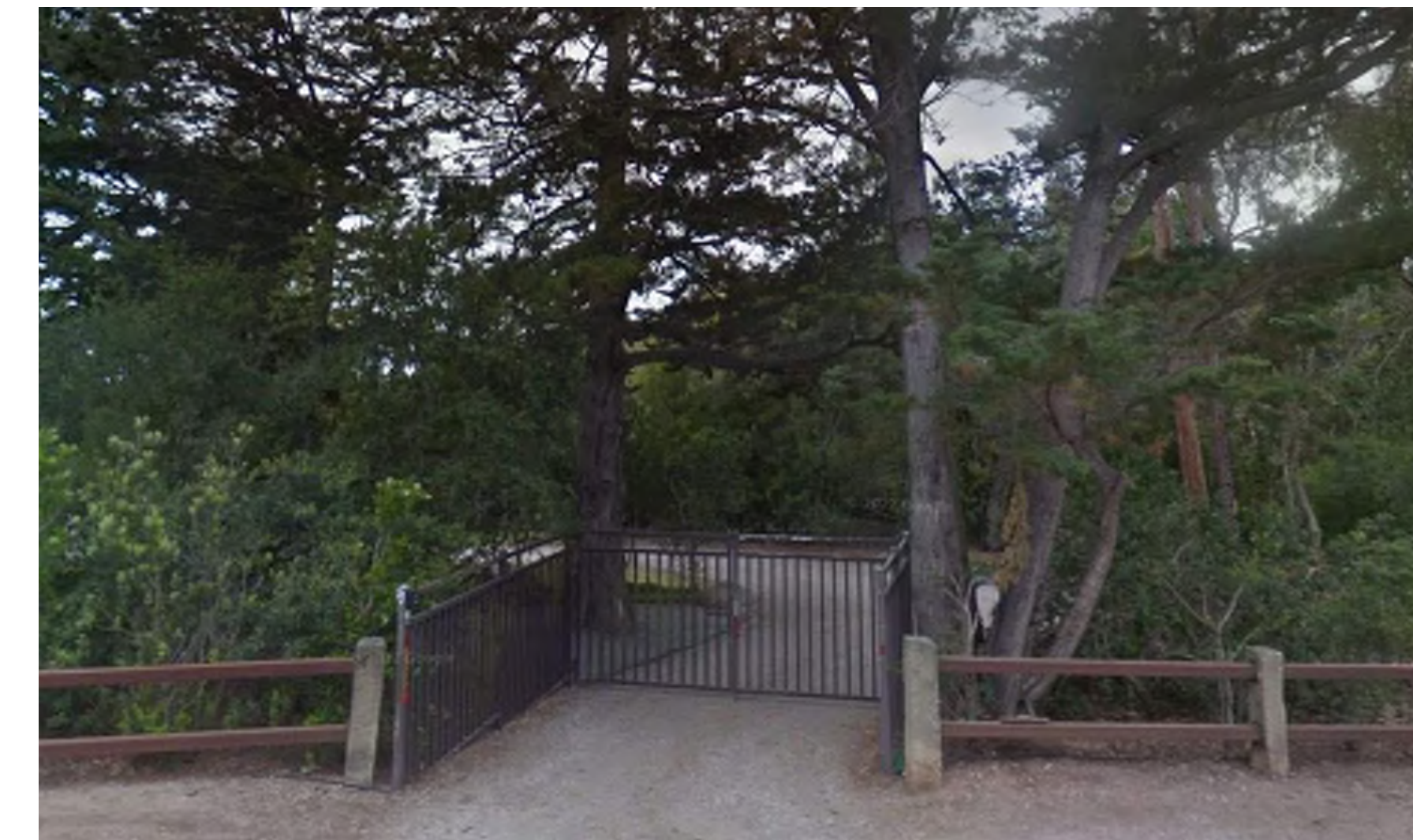
12. Entry gate at guest house
