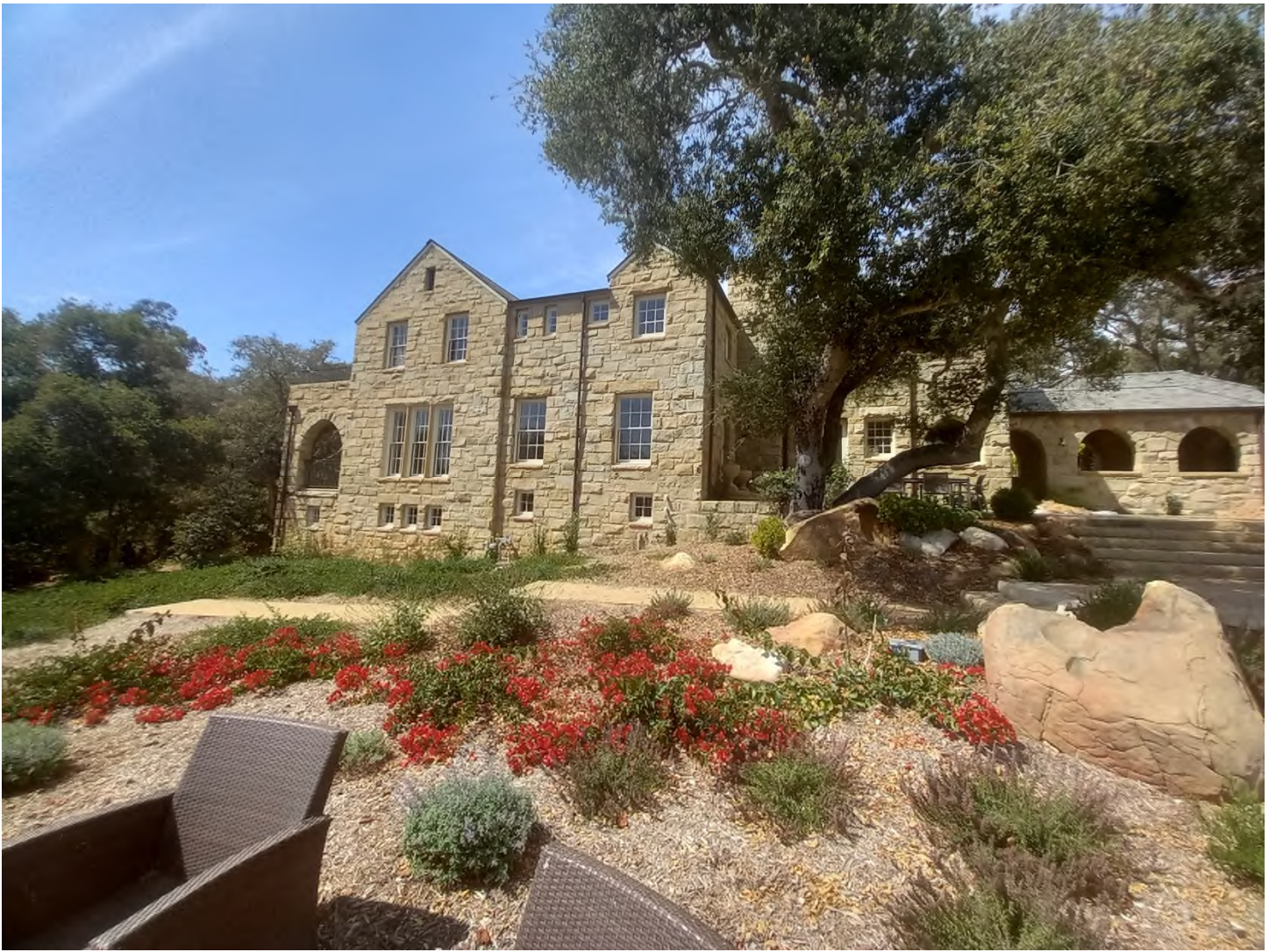
Photograph 9, Residence, south elevation, looking north
