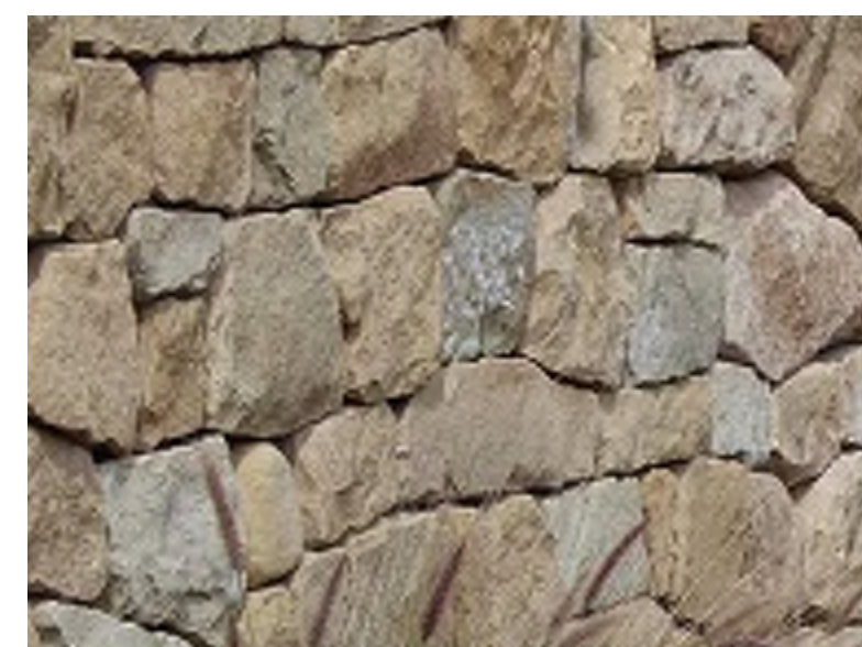
Cut stone to match (E) stone wall
