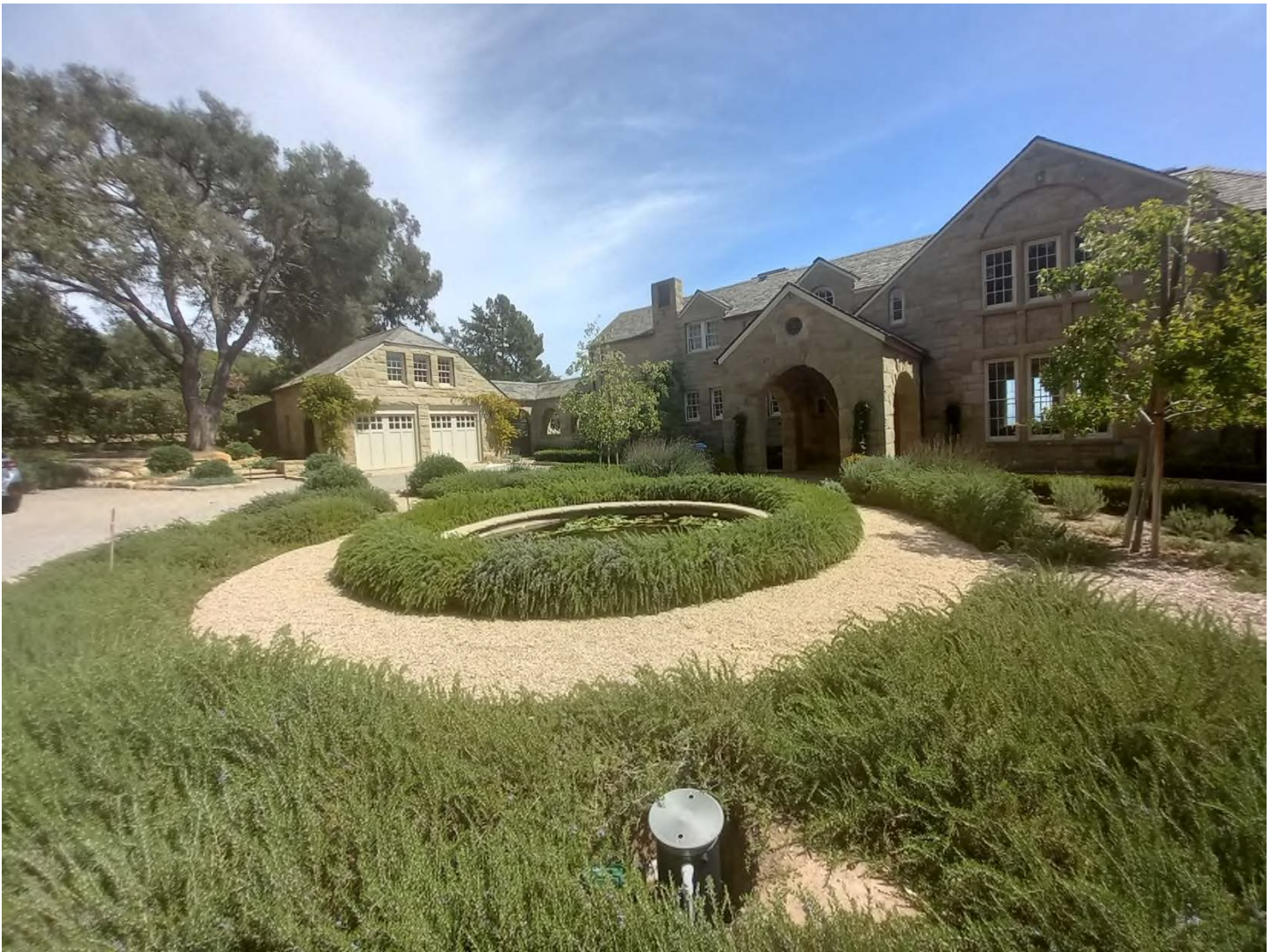
Photograph 2, Residence, Garage, and Motor Court, looking southeast
