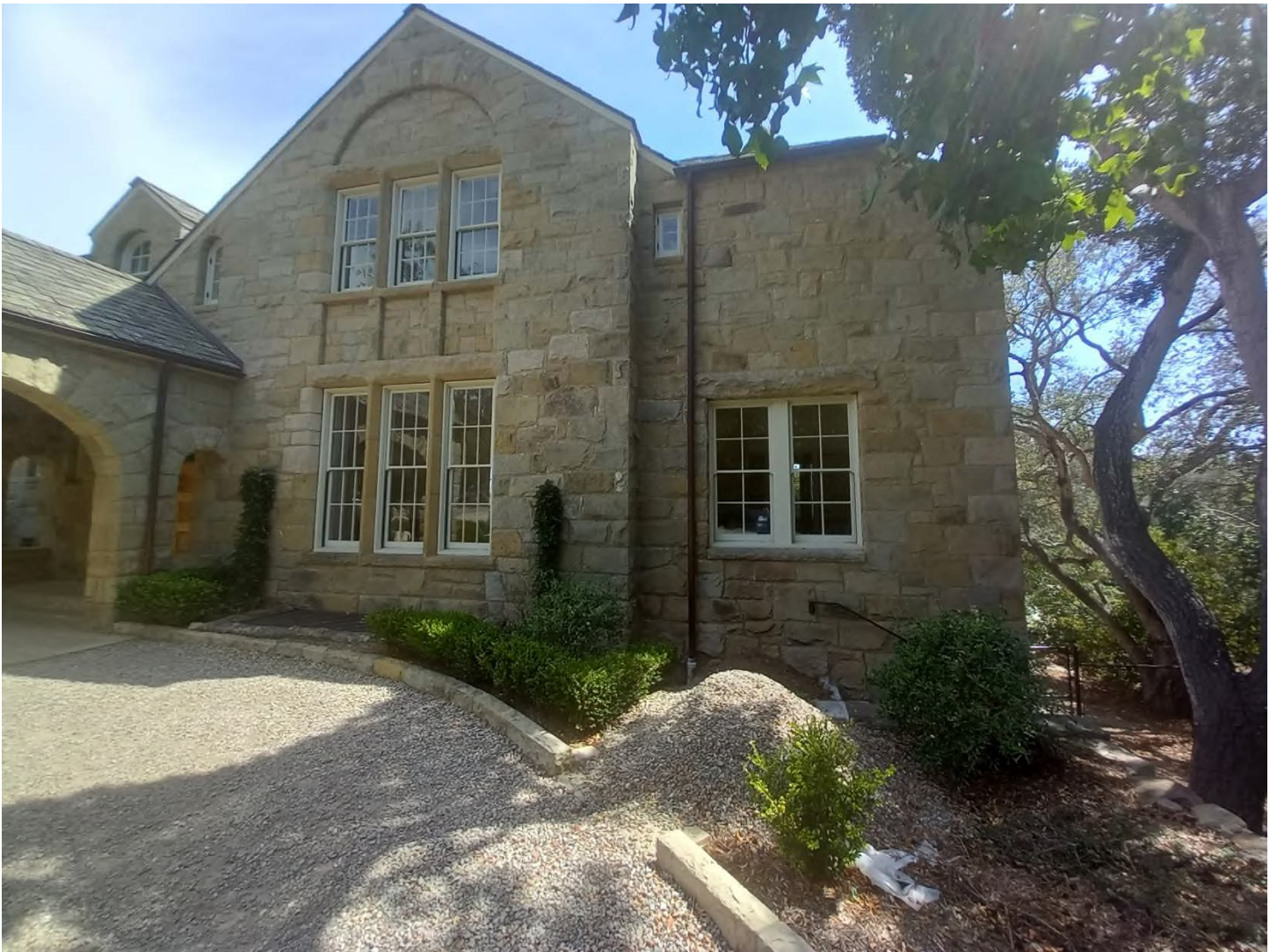
Photograph 4, Residence, west end of the north elevation, looking south
