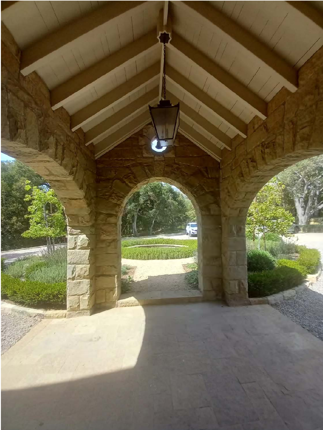
Photograph 6, Residence, Looking north from the porte-cochere to the motor court
