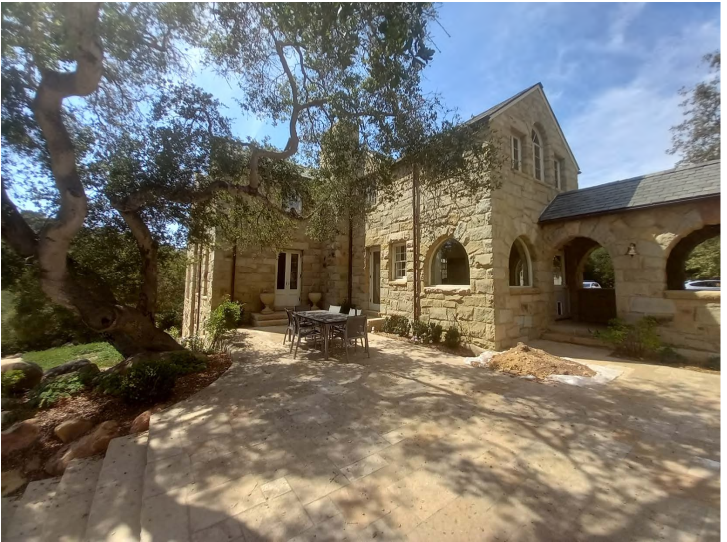
Photograph 16, Residence, East elevation, looking northwest
