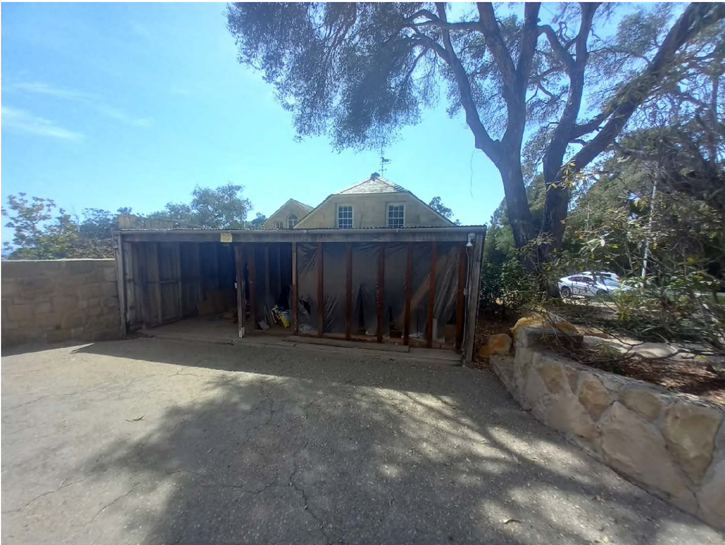
Photograph 17, Garage, East elevation, looking west
