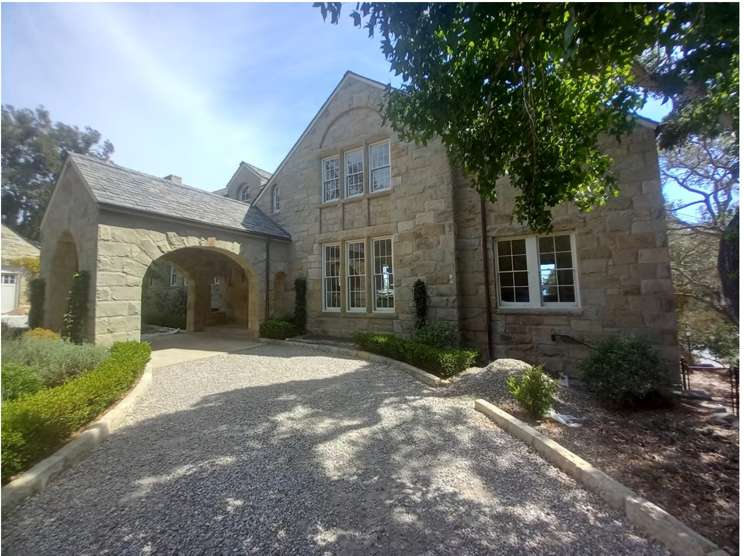
Photograph 3, Residence, west end of the north elevation, looking southeast
