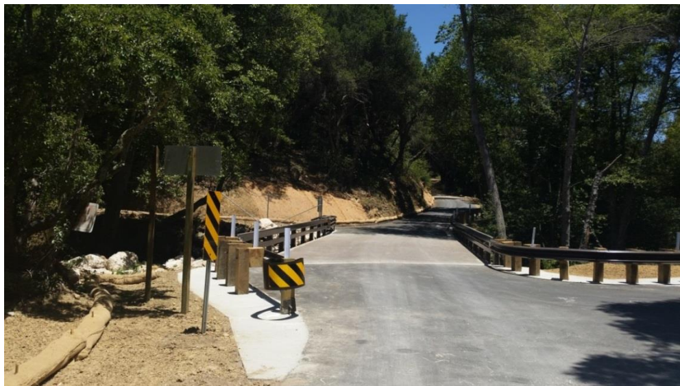
New Kinevan Road Bridge No. 51C-0372 over San Jose Creek
