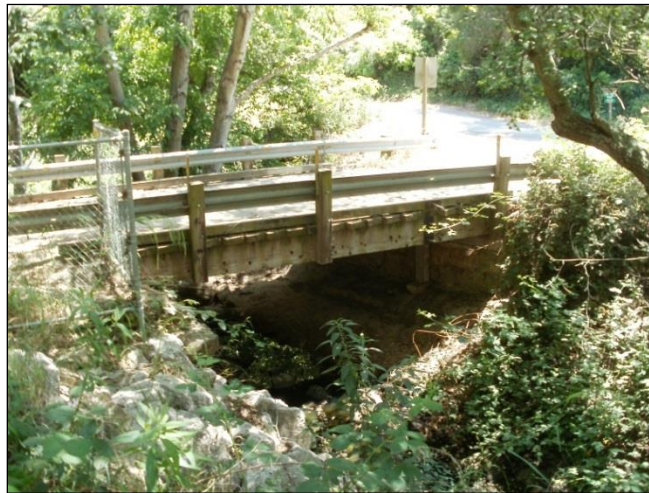
Previous Kinevan Road Bridge No. 51C-0214 over San Jose Creek
