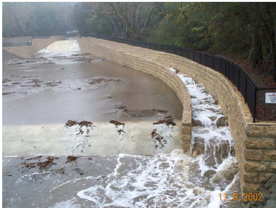
Montecito Creek Debris Basin on November 8, 2002
