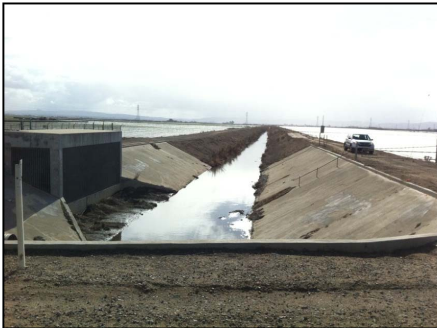
Figure 2.2-4. Northern Portion of Unit 2 Channel (looking southward)
