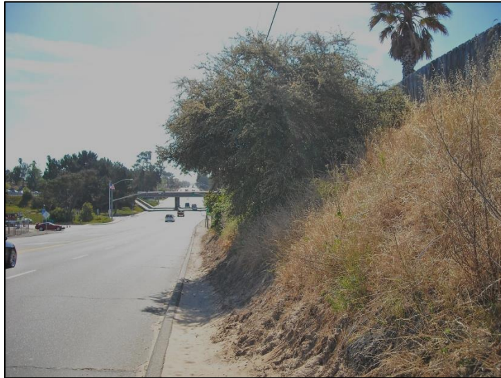
Clark Avenue, view towards State Route 135
