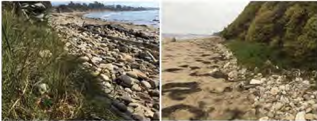
Example nature-based solution: Constructed cobble berm in Goleta (left) and Arroyo Burro Beach (right) dissipating wave energy and erosion and creating habitat from Newkirk et al. Toward Natural Infrastructure to Manage Shoreline Change in California (2018)
