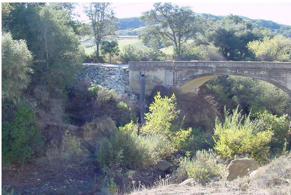
Photo: Existing Bridge 51C-113
