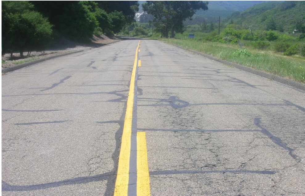
Miguelito Rd, typical to be rehabilitated
