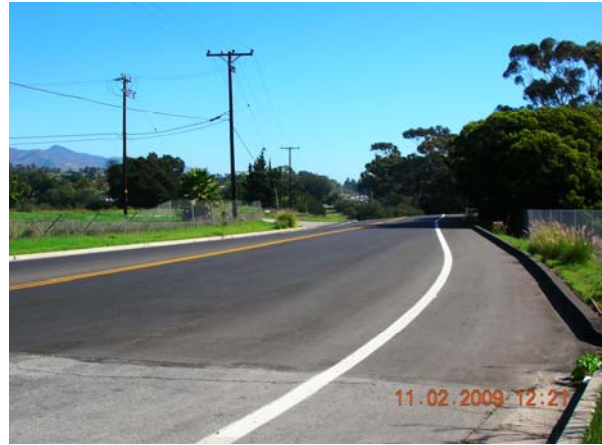
Calle Real After
