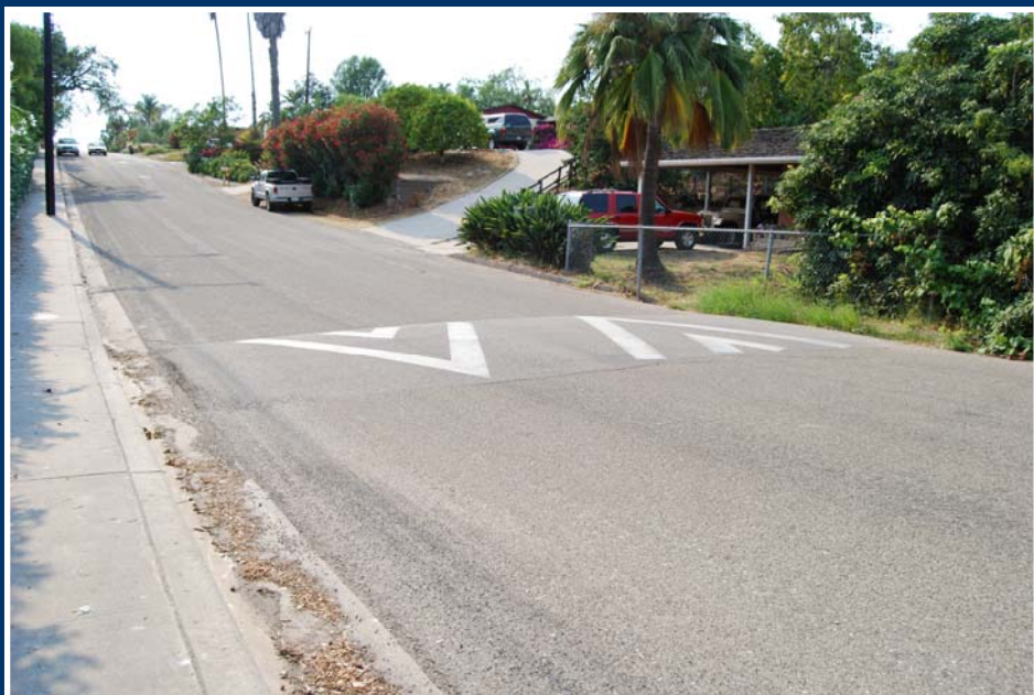
SPEED HUMP – PUEBLO AVENUE
