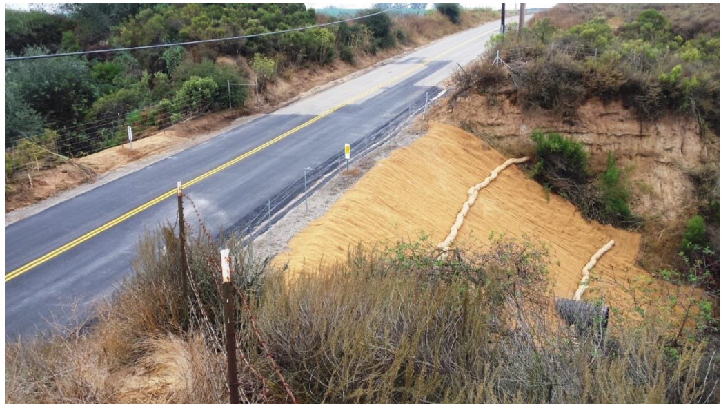
September 5, 2017 - Construction complete
