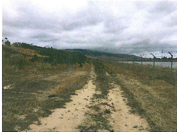
b. Soil stockpile (left), new supply line alignment (center) and reservoir (right)
