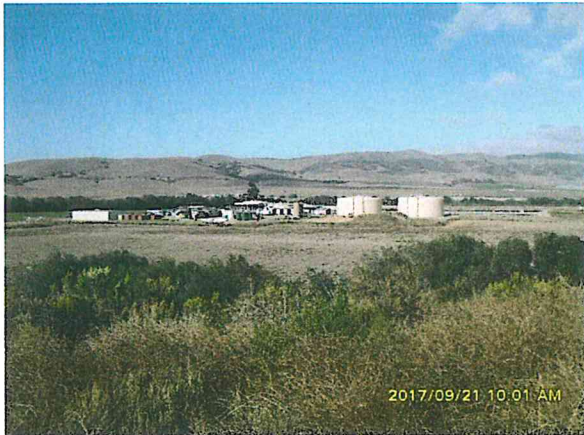
a. Phase 1 WWRP Upgrade site (center) adjacent to existing WWRP
