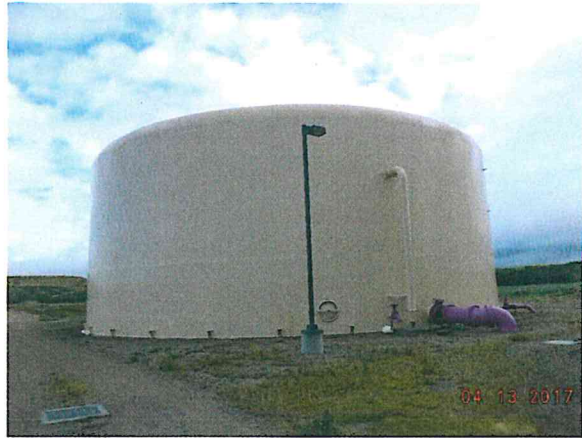
d. Example of the tank to be constructed at Waller County Park
