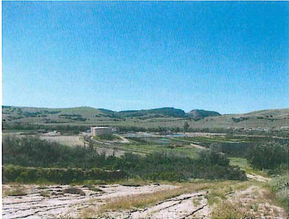
a. Wastewater Reclamation Plant from near the reservoir soil stockpile
