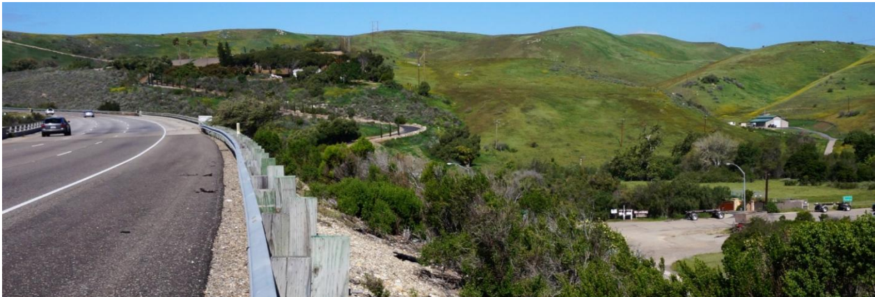
Fig. 8.3- Intrusion: Residential home and barn visible looking north at PM 36.50 as drivers cross Refugio Canyon.
