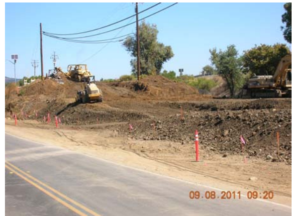
Excavation for Embankment on Santa Rosa Road
