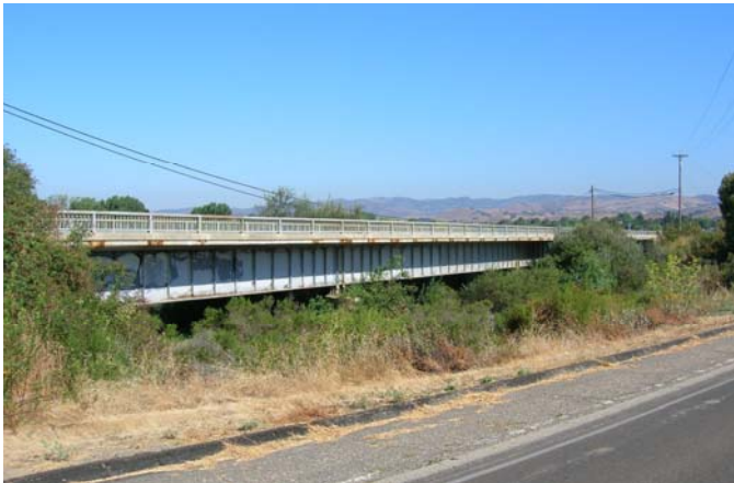
Bridge 51C-173 on Santa Rosa Road
