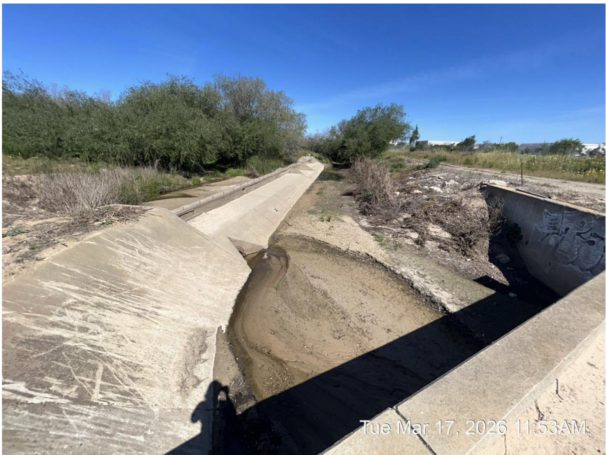
Santa Maria Airport Ditch Section 1
