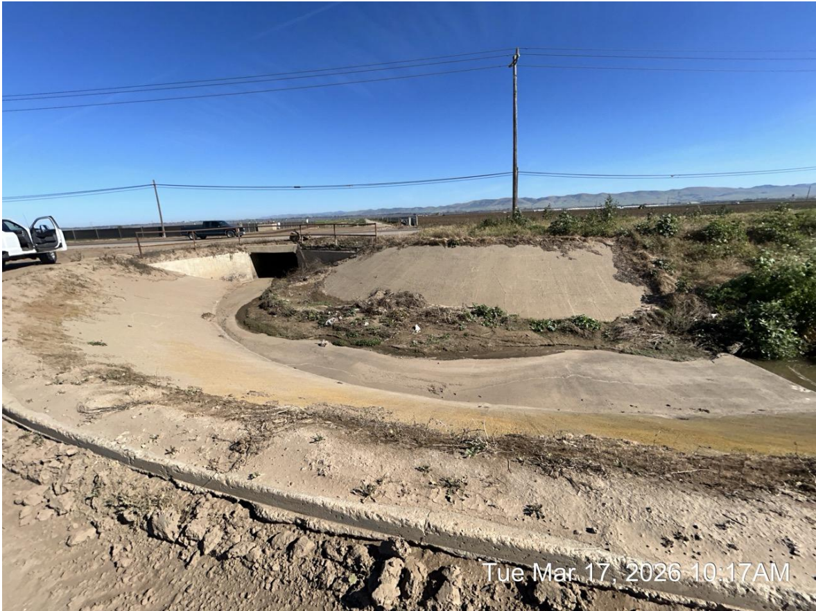
Unit 2 West Main Channel Section 3
