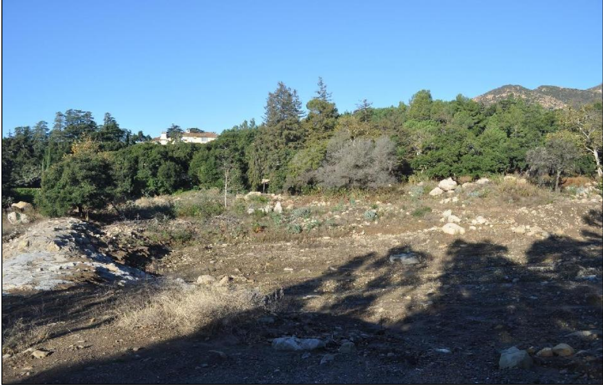
Photo 1. Existing Debris Basin Dam Embankment and Expansion Area
