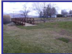
Pedestrian bridge Richardson Park
