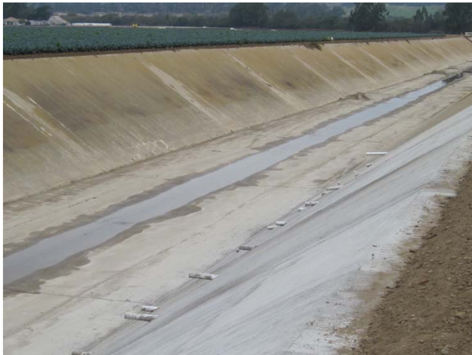
Rodeo- San Pasqual Repair Project Completion
