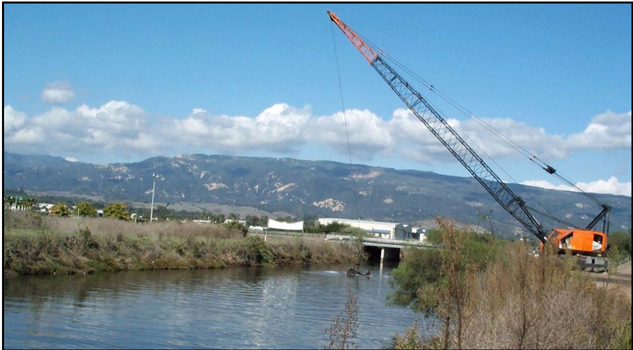
Figure 2-6. Dragline Desilting
