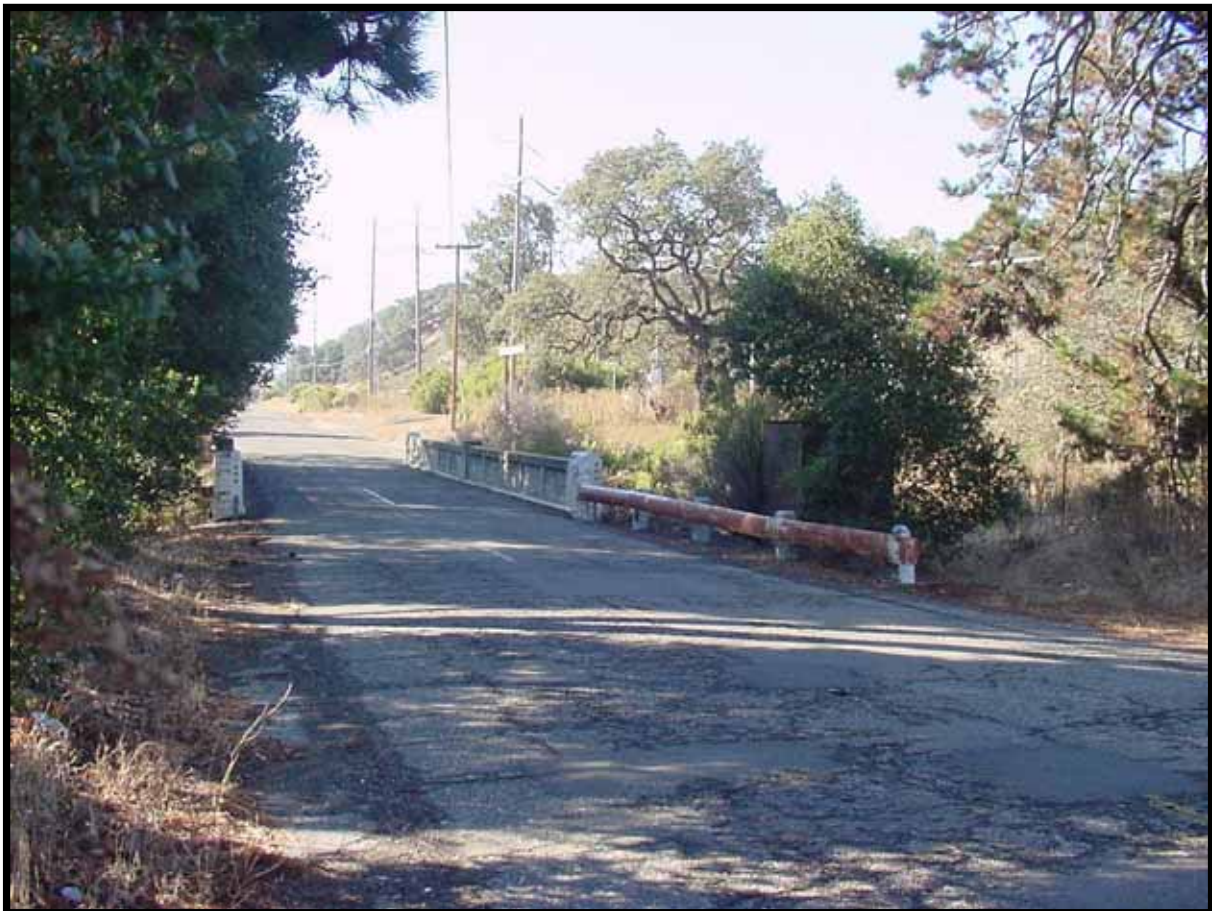
Existing Bridge No. 51C-0225, looking south on Jonata Park Road
