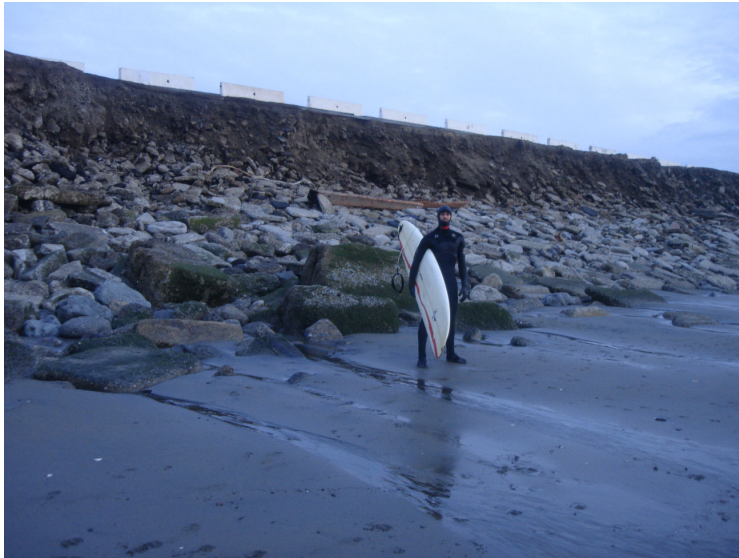
Figure 3: Picture(s) of existing rubble, SOB. Photograph © Bob Battalio, taken February 1, 2010.
