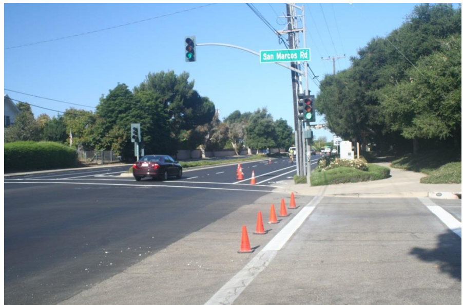
Hollister Avenue at San Marcos Drive after striping
