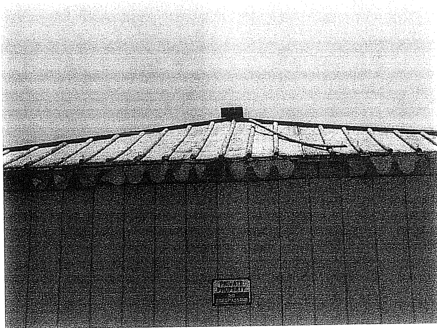
Plate 14. Beach house showing sheet metal scallop detail and original walls beneath protective plywood paneling. Facing east. A. C. Cole, July 2001
