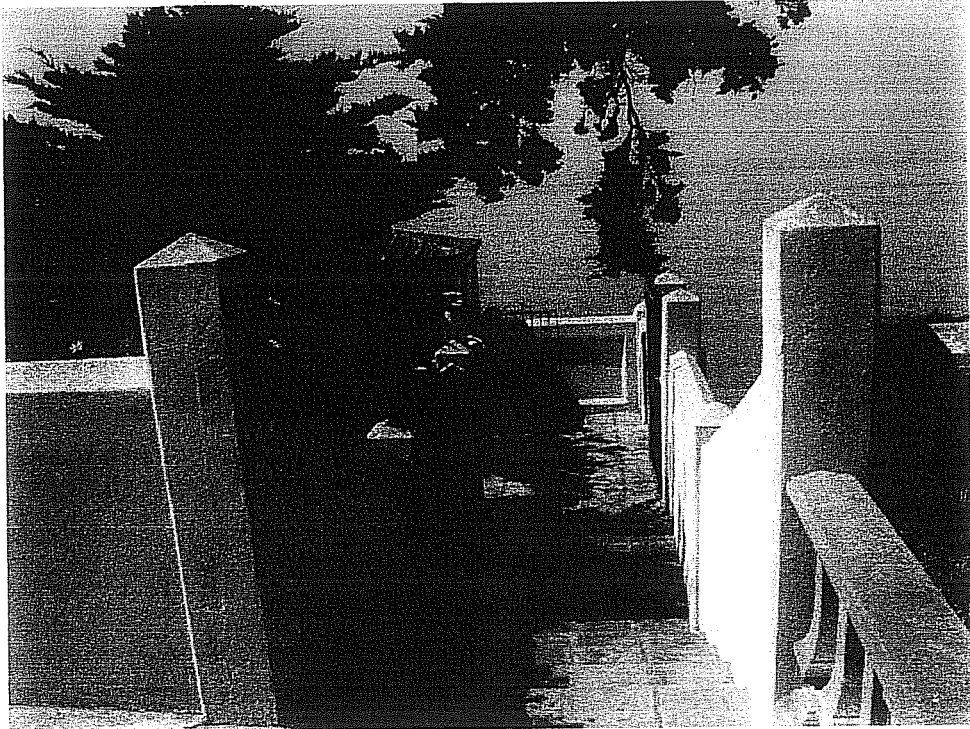
Plate 7. Entrance steps to elevator platform. Facing south. A. C. Cole, July 2001
