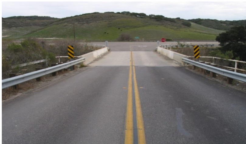
Existing Jalama Road Bridge 51C-013 – Looking East
