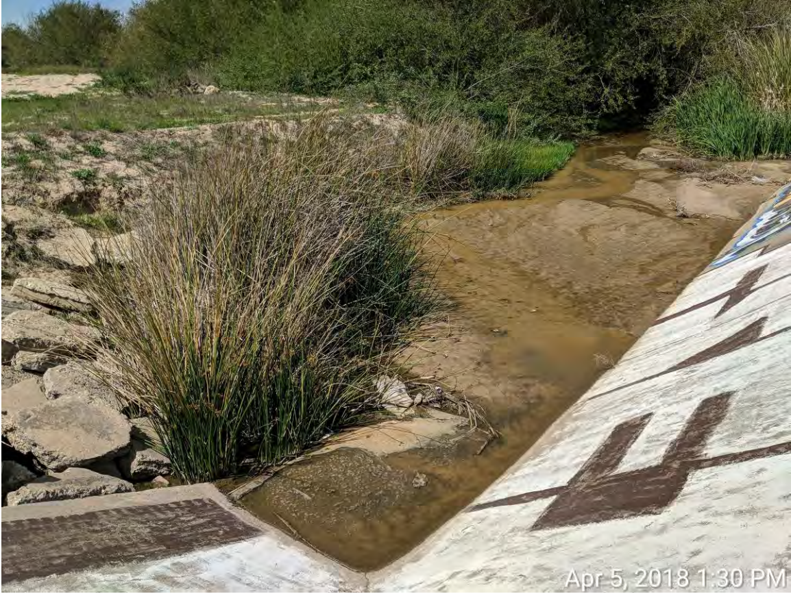
Santa Maria Airport Section 3
