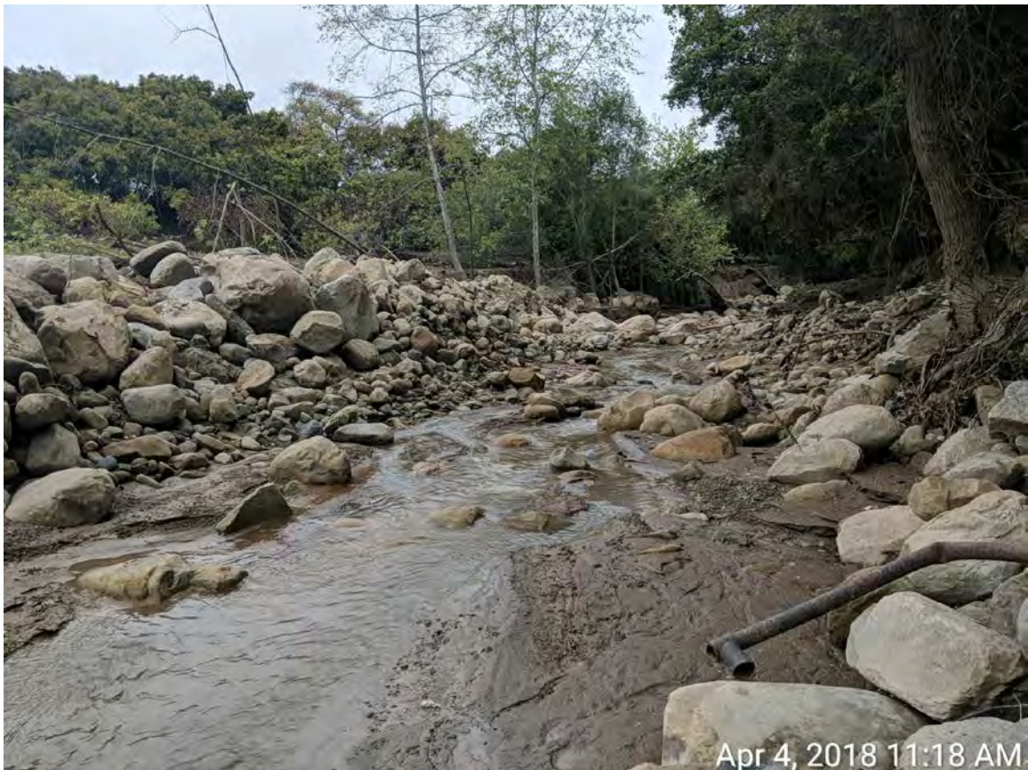
Section 7 (Looking upstream)
