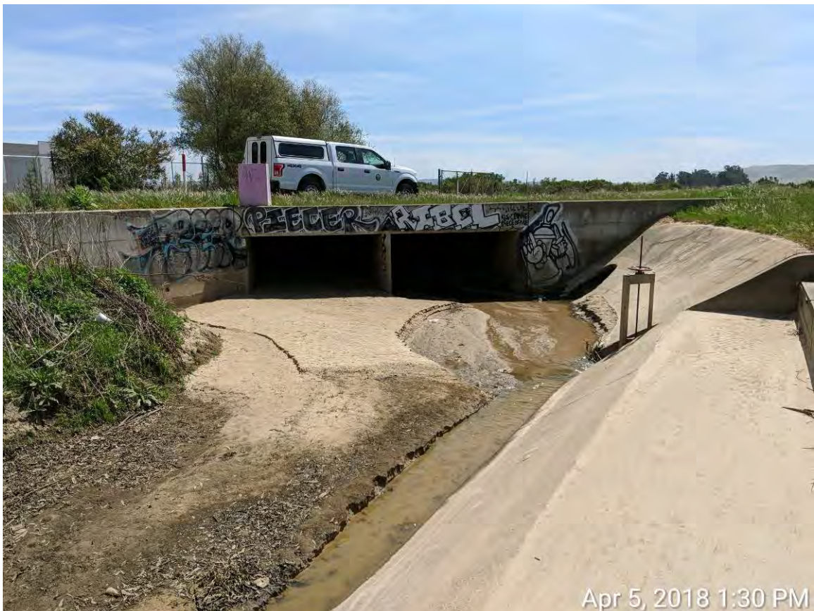
Santa Maria Airport Section 2
