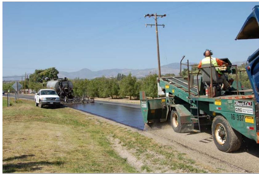
Typical scrub seal operation on a rural road
