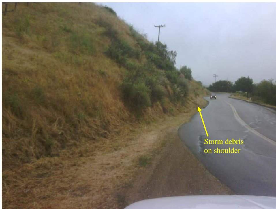
San Marcos Road – Existing Conditions (Looking North)
