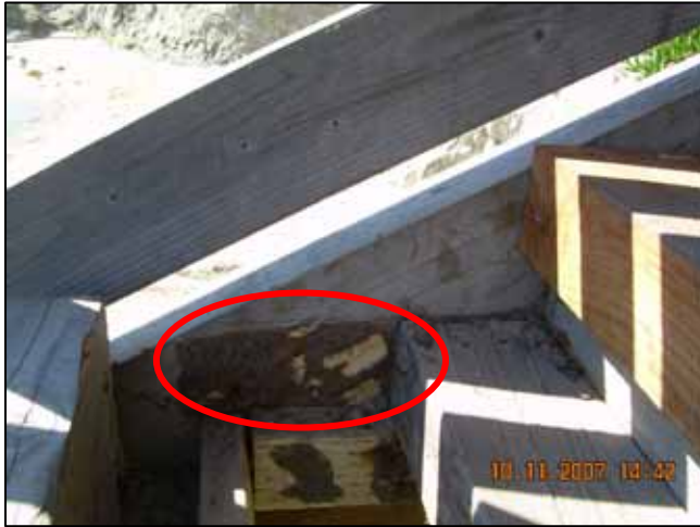
Termite and dry rot damage revealed after disassembly of stairway elements
